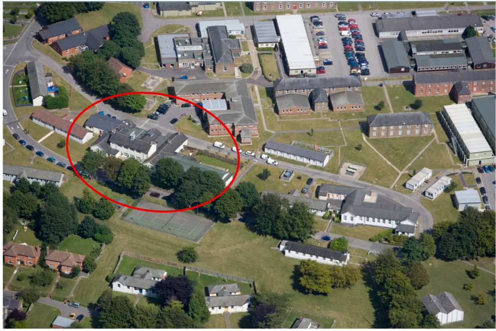
Avon Club, Sergeants' Mess, Building 110 (circled) (Perspective Aerial)
