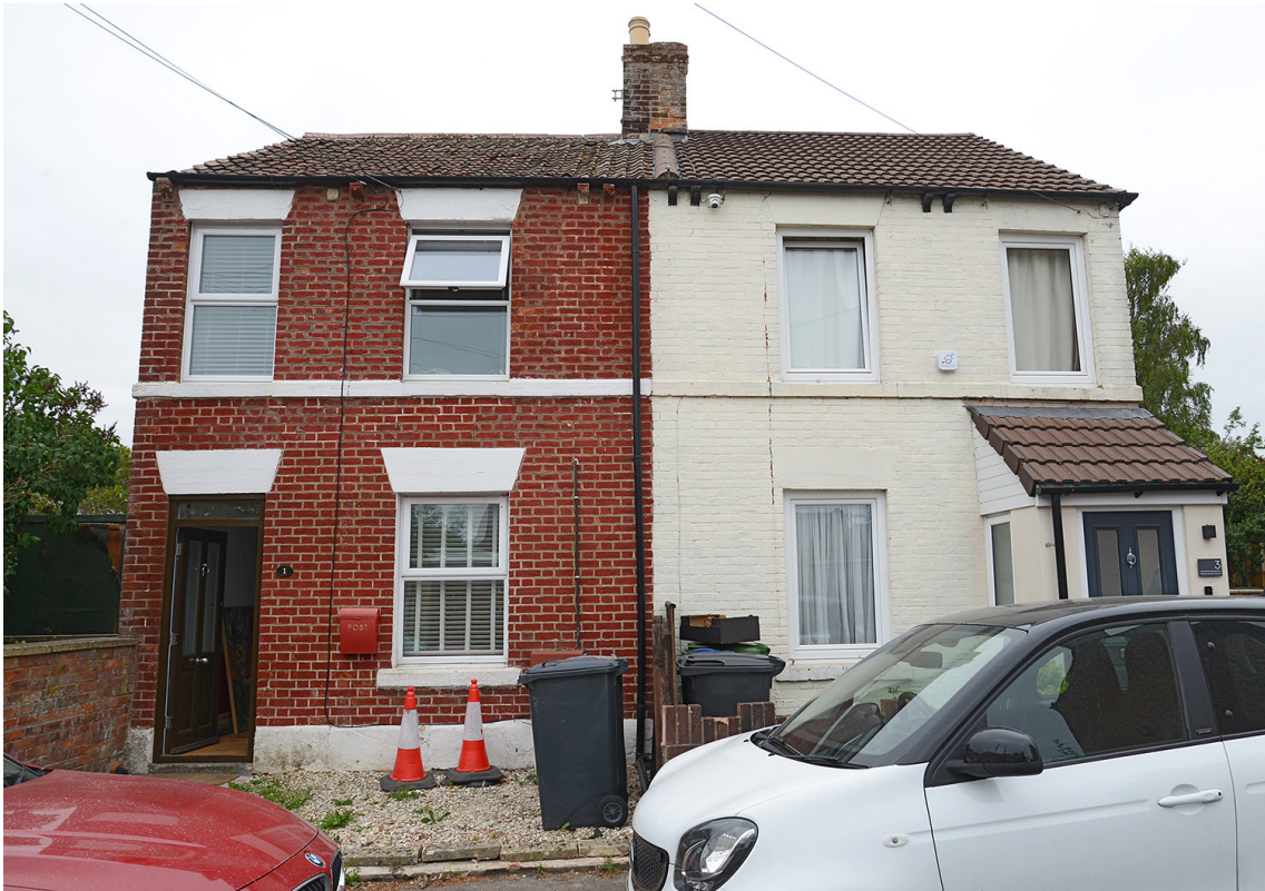
FRONT OF EXISTING PROPERTY FROM THE ROAD
