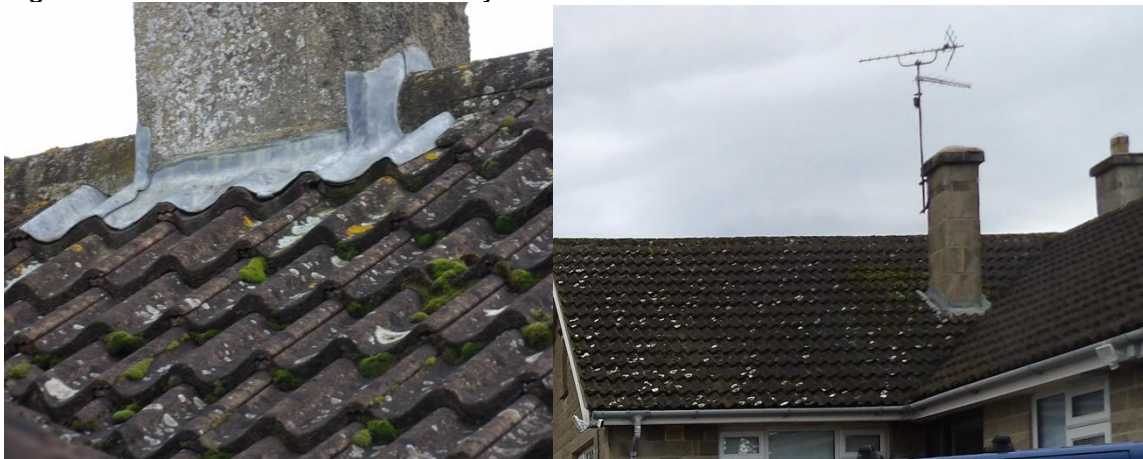
Figure 7/8. Leadwork around chimneys.
