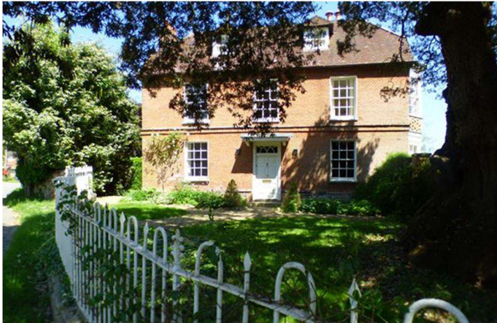
WOODFORD UPPER WOODFORD SU 13 NW (east side) 8/269 Shepherd's Close and front railings
