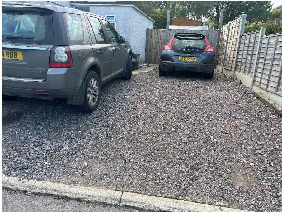
Photograph 2 – The hardcore driveway to the front of the property
