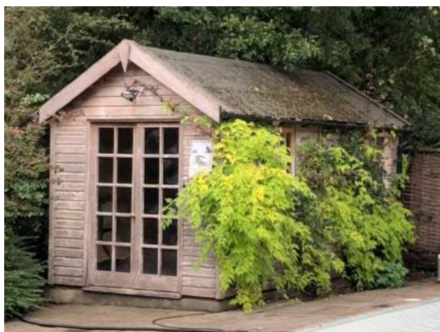
Image 6: Plant growth and window on the western side of the shed
