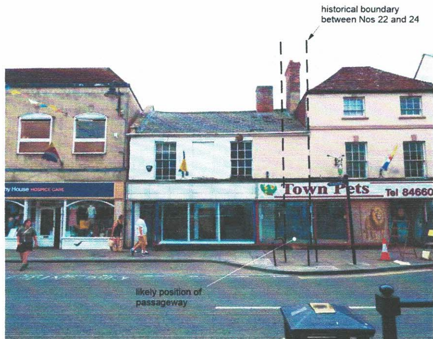
North elevations of Nos 22 and 24
