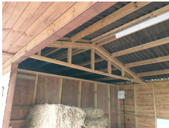
Figure 8: Internal view of the stable building.
