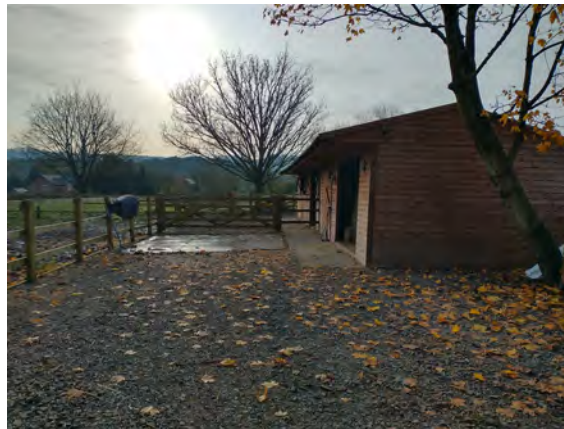
Figure 1: Gravel surface north and east of the stable building.
