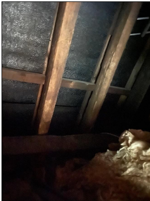
Picture 3: Inside the roof where the solar slates are proposed
