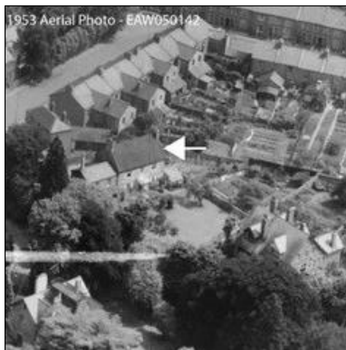
Picture 6: 27 Langley Road in 1953
