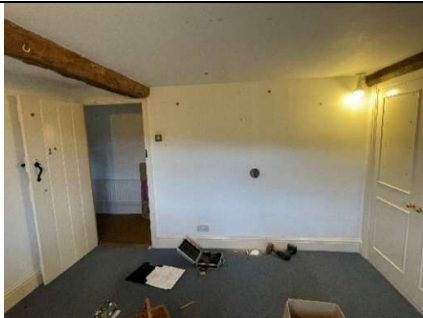
Modern partitions in Bedroom 02 + Door 2 to be re-positioned
