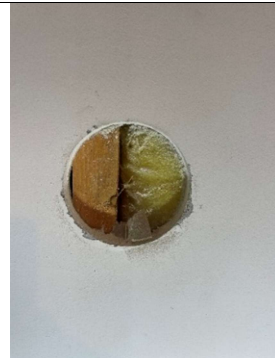
Plasterboard and timber studs
