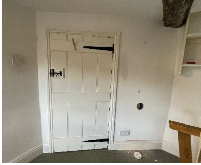
Modern partition in Bedroom 03 + Door 3 to be re-positioned
