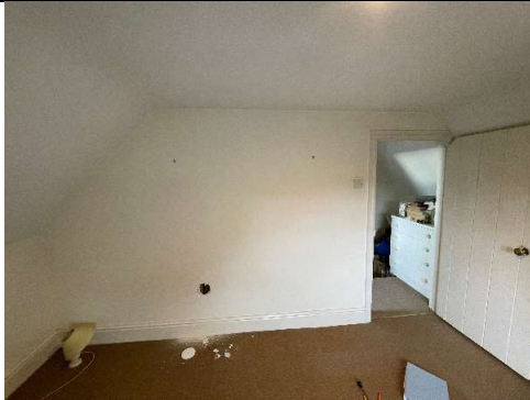
Modern partition in Bathroom 03
