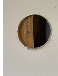
Plasterboard and timber studs
