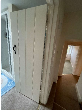
Existing modern door removed
