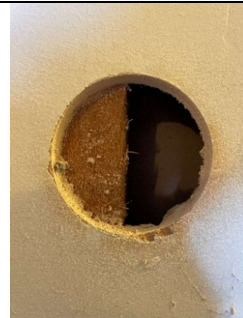
Plasterboard and timber studs
