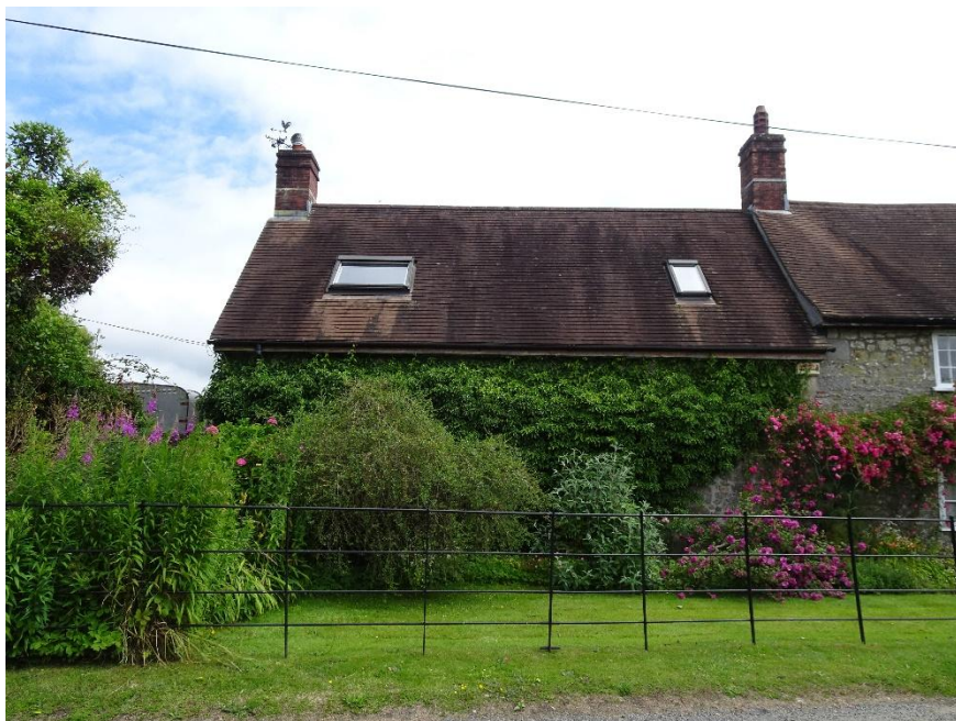
Previous outbuilding (now reception 01) attached to north-west gable of farmhouse
