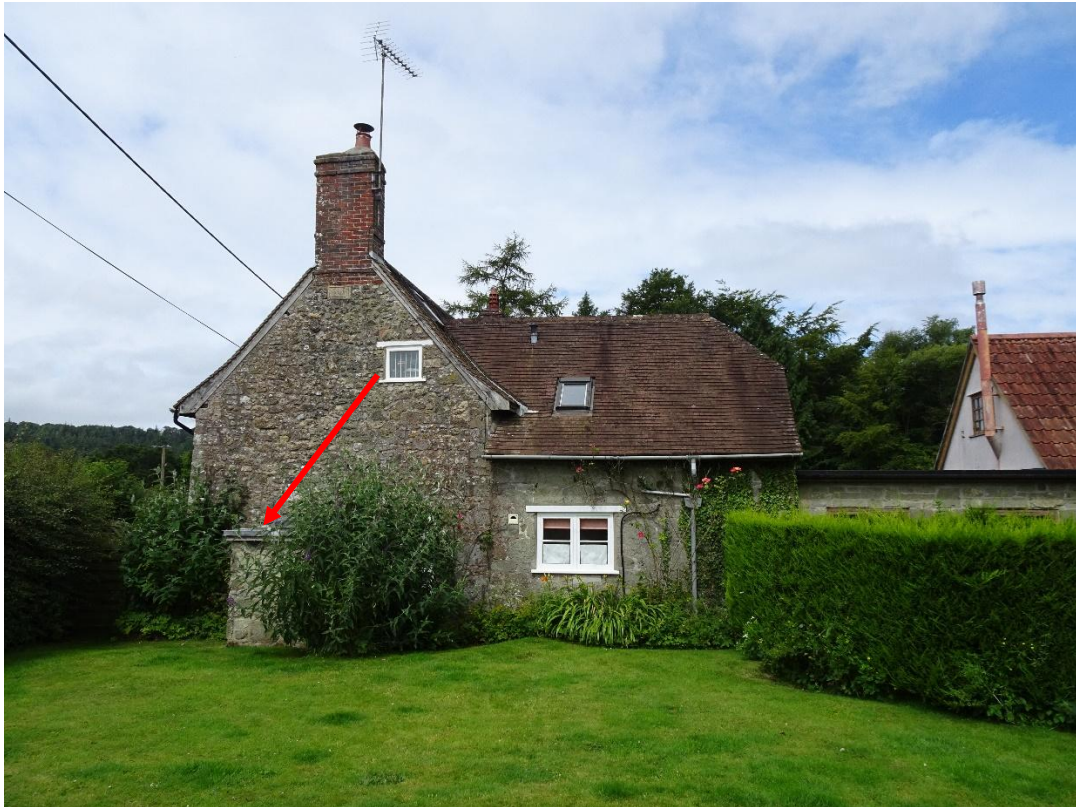
South-east gable of farmhouse with modern boiler room. Red arrow indicates modern boiler room.
