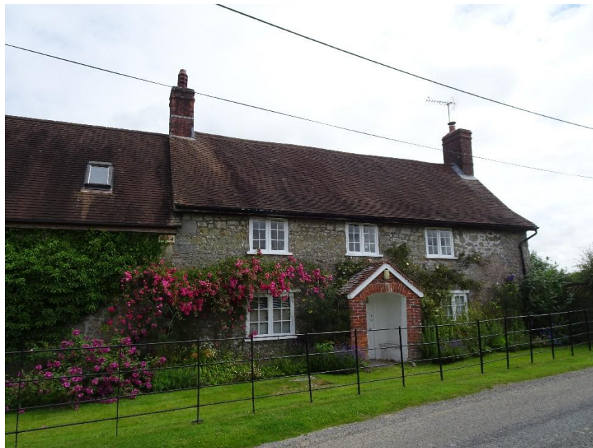
Front (south-west) elevation of farmhouse with previous outbuilding (now reception 01) attached to north-west gable
