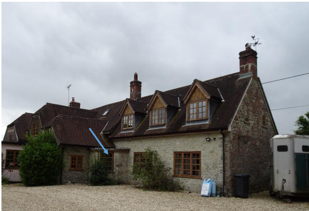
Rear of farmhouse (from north). Blue arrow indicates window set within 1995 wall (LBC S/1994/1835).
