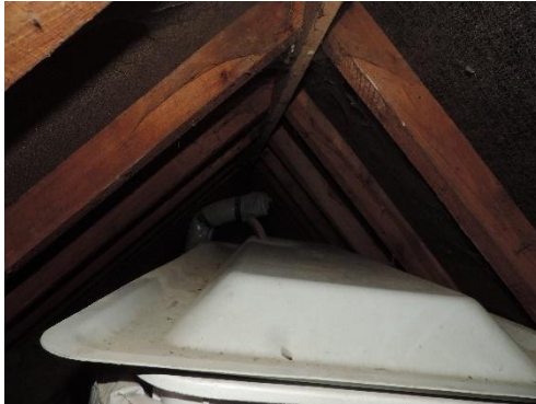
Plate 5: Section 2 Loft Void
