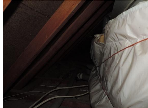
Plate 6: Section 2 Loft Void
