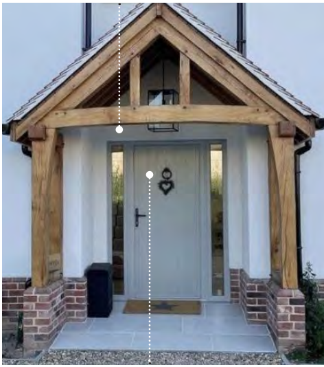
Traditional style timber framed porch on rustic brick plinth
