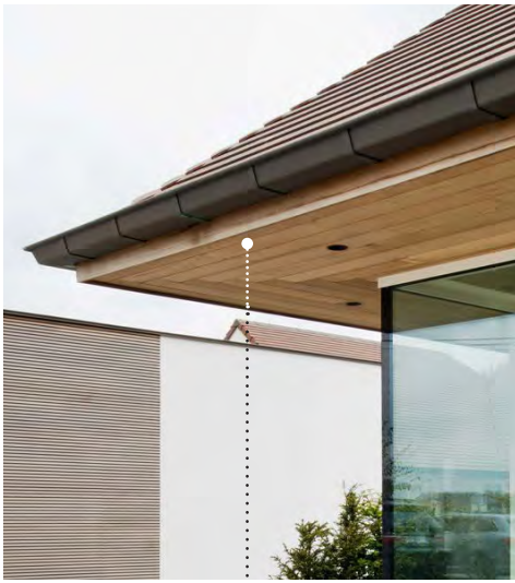
Overhang/canopy for solar shading
