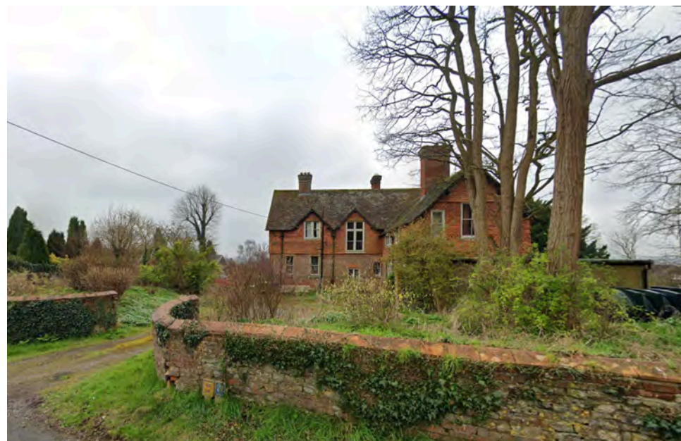
View of The Old Vicarage North Elevation from Little London Road.
