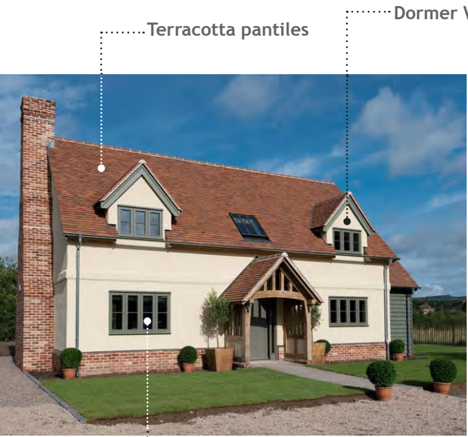
Flush casement painted timber windows
