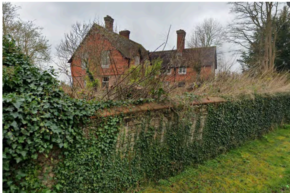
View of The Old Vicarage East Elevation from Little London Road.
