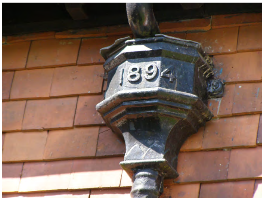
Plate 3. Cast iron rainwater head from Old Vicarage, dated 1894, the date the building was constructed
