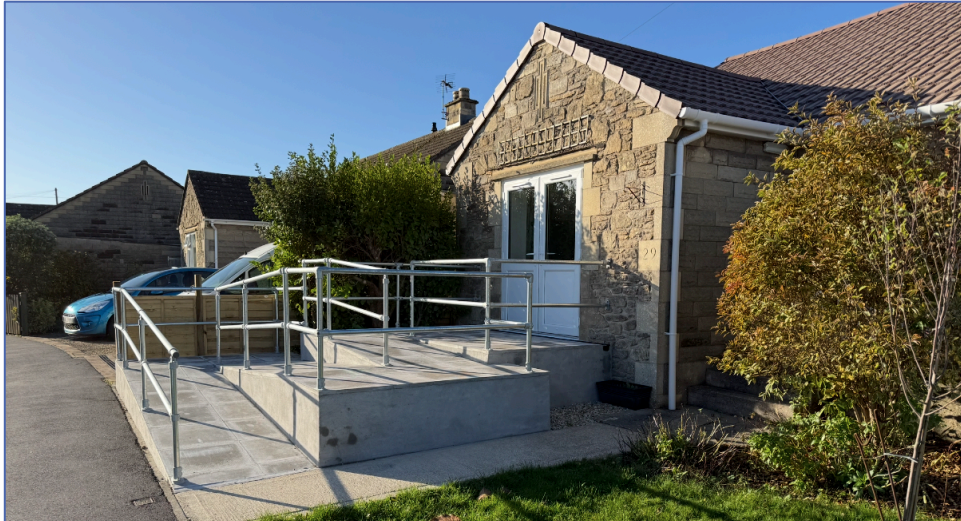
Figure 6. Photograph of the recently installed ramp, taken from the public footpath to the north of the site.
