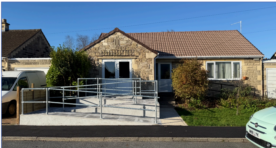
Figure 7. Photograph of the recently installed ramp, taken from the east.
