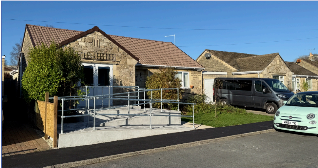
Figure 1. Photograph of the application site, showing No.29 and the recently installed compliant ramp which provides access from the front bedroom to the public footpath and highway.
