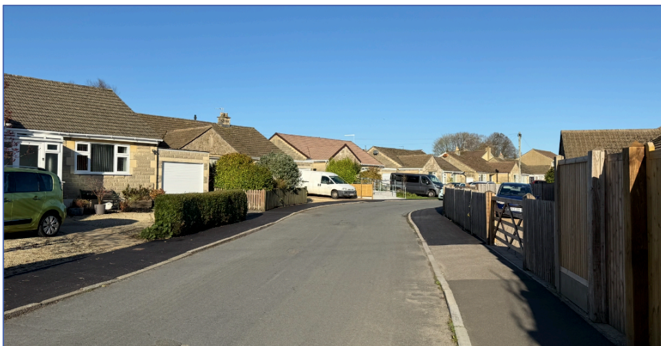
Figure 8. Photograph of the recently installed ramp, shown in the context of the street scene.
