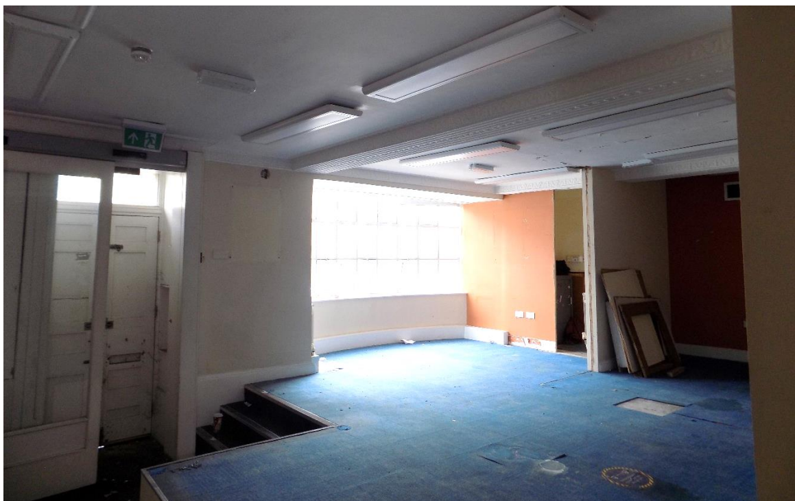
Fig.15: Ground-floor frontage range internal view, showing moulded beams and raised floor.
