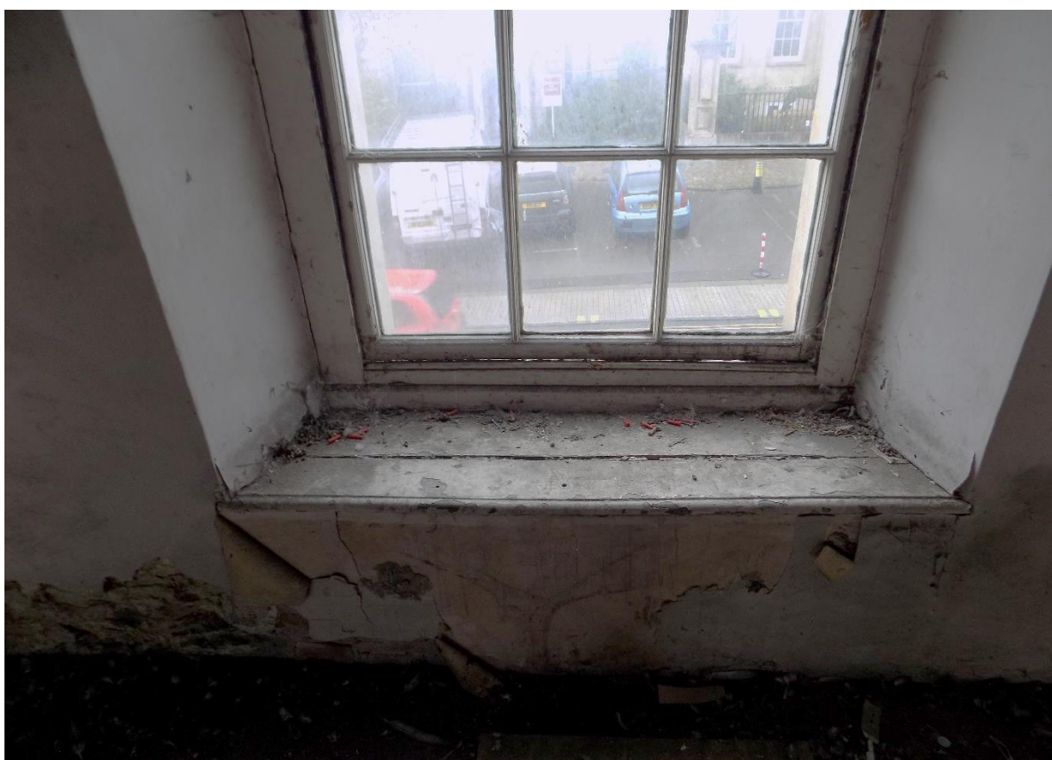
Fig.27: First-floor: Detail of second front-facing window from west, showing historic window sill.
