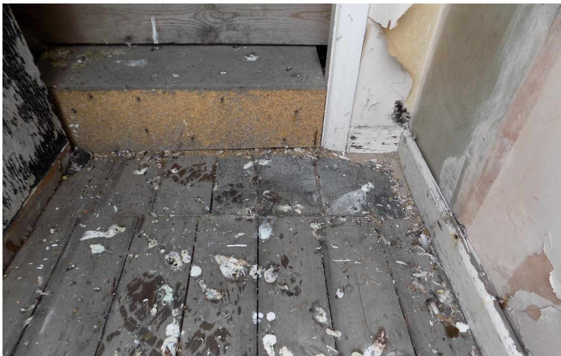
Fig.24: First-floor lobby detail, showing two oak floorboards disappearing under the false floor .
