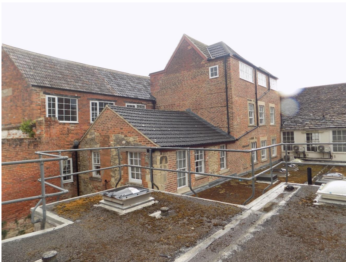
Fig.57: View looking south-west from the location of the proposed four-story block, showing the four-storey building to the rear of No.2 Fore Street. This formed the rear service wing to the combines Nos 2 and 3 Fore Street. It has been extended in height in, at least, two phases.
