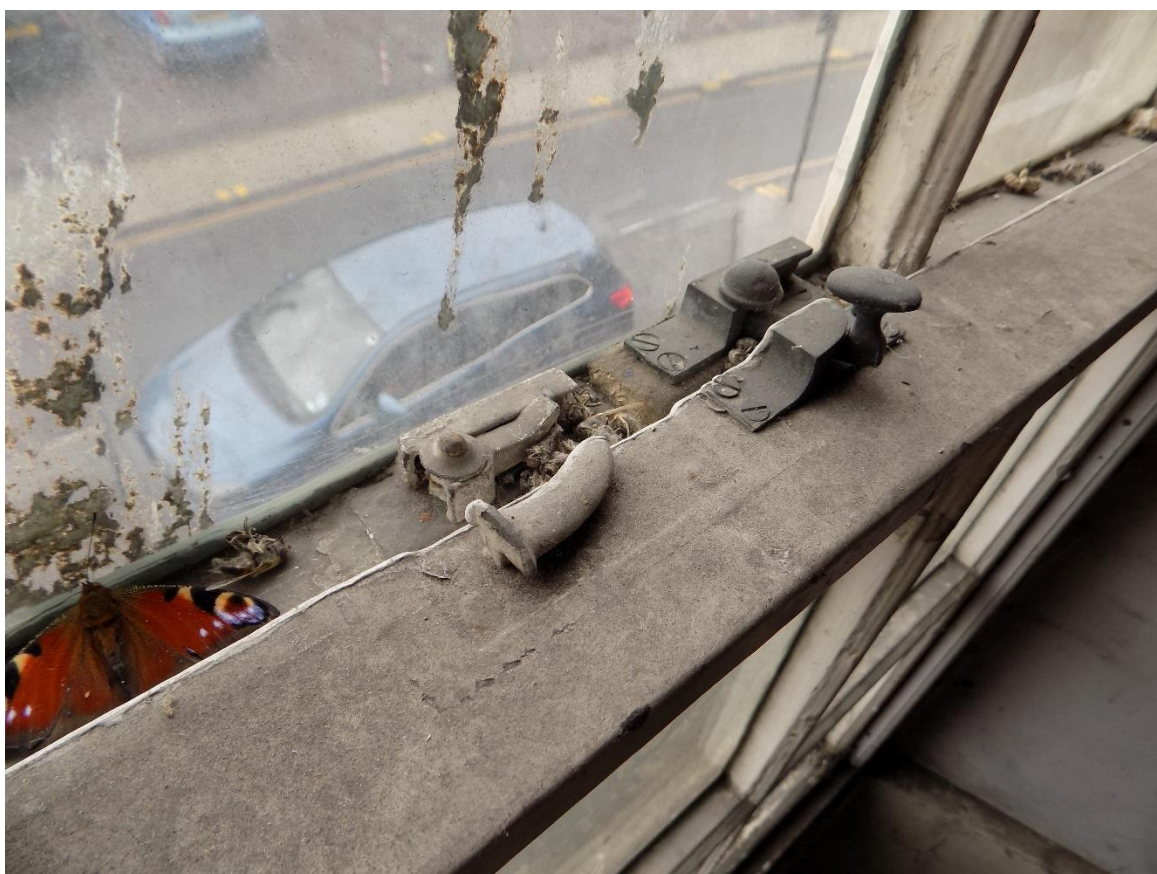
Fig.33: Window detail, showing window catch and early twentieth-century replacement.
