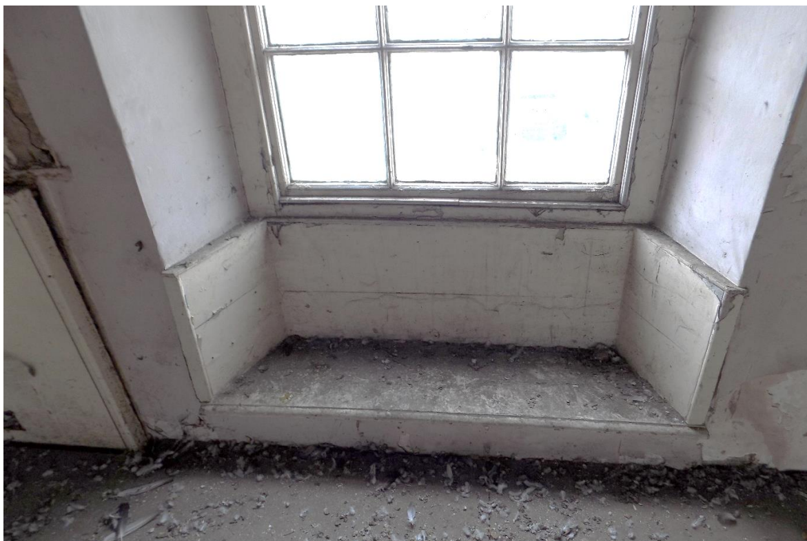
Fig.26: First-floor: Detail of first front-facing window from west, showing historic window seat truncated by false floor.
