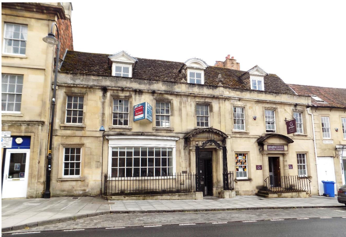
Fig.8: Contemporary view showing No.2 Fore Street (to right) following the removal of the Victorian shopfront and addition of central, pedimented door in stone.
