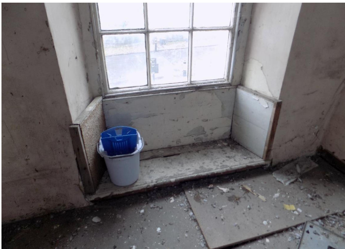
Fig.29: First-floor: Detail of fourth front-facing window from west, showing historic window seat truncated by false floor.
