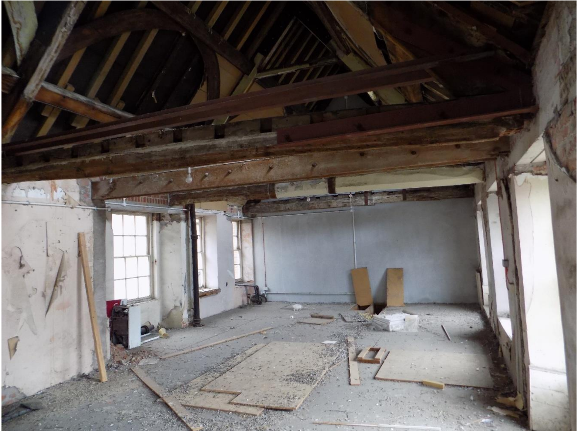
Fig.22: General view of the first floor, looking south-west, showing suspected chimney-breast and recessed window to left.
