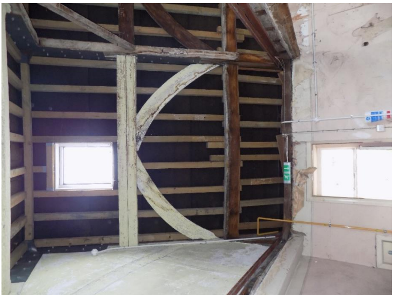
Fig.46: Views of underside of south slope of roof, showing curved wind-braces and extensive replacement of rafters.
