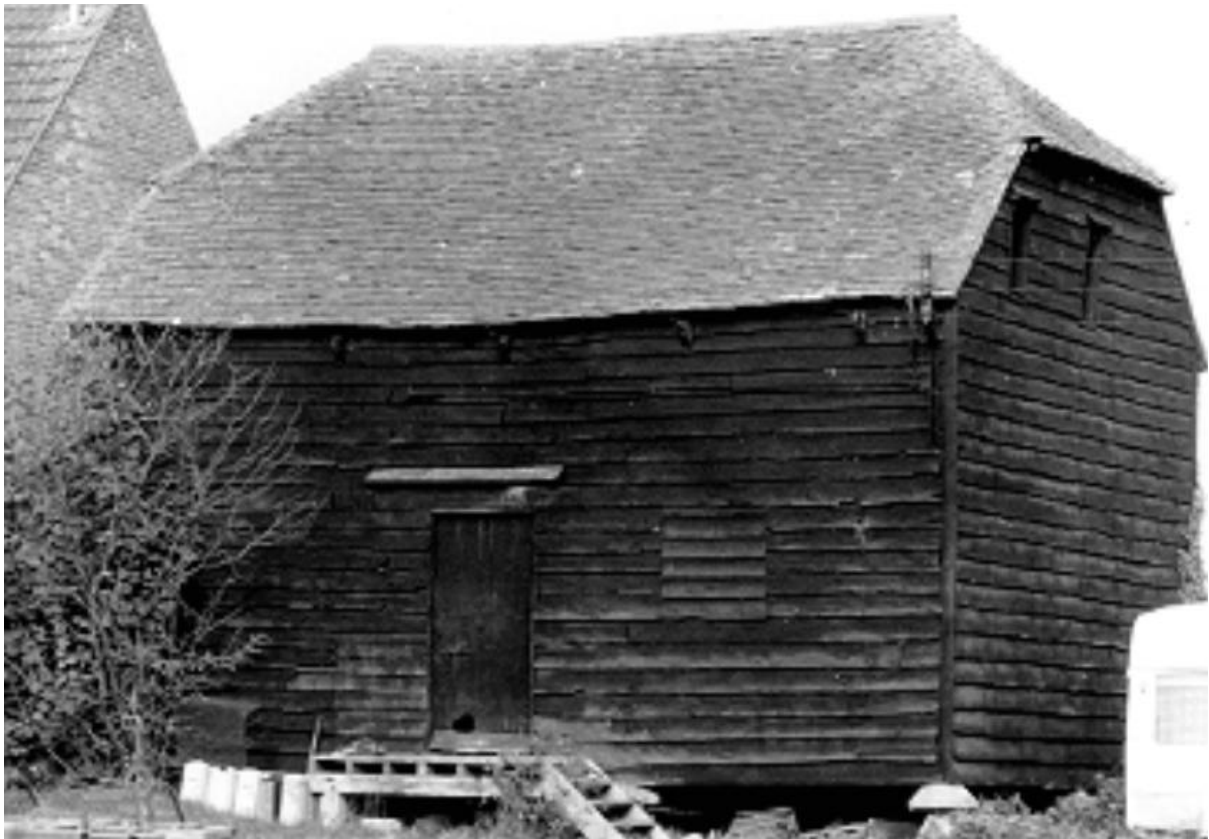
Figure 3 - East elevation from National Trust Vernacular Building Survey 2000
