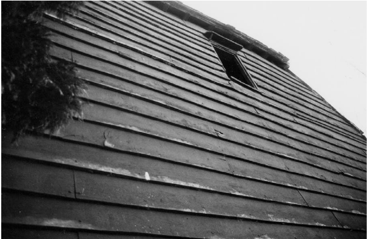
Figure 4 - South Elevation timber boarding from Vernacular Building Survey 2000
