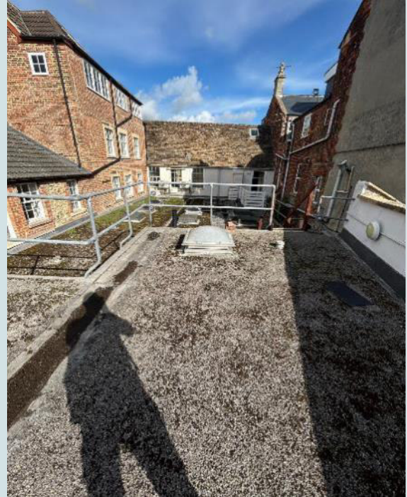
Southern elevation viewed from the south looking north
