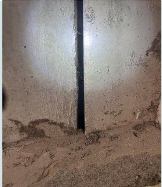
Cavity is created by the double concrete window lintels
