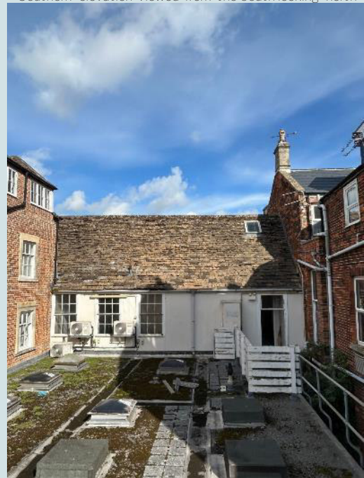
Southern roof elevation and first southern extension flat roof
