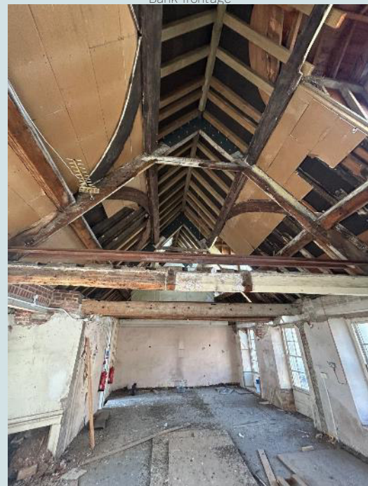
First floor internal space
