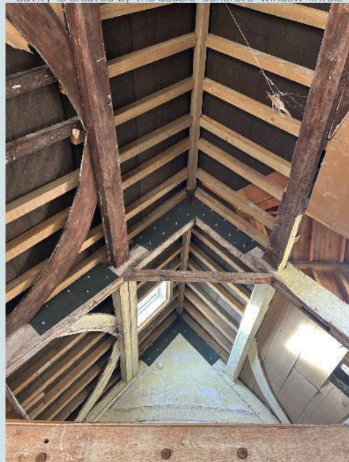
Cut roof A frames and bitumen felt, also showing the bracing on the roof.
