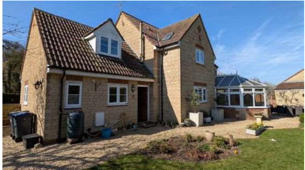
2 - View of rear existing
