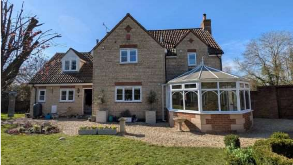
1 - View of rear existing
