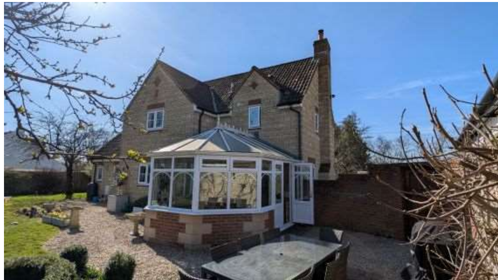
3 - View of rear existing
