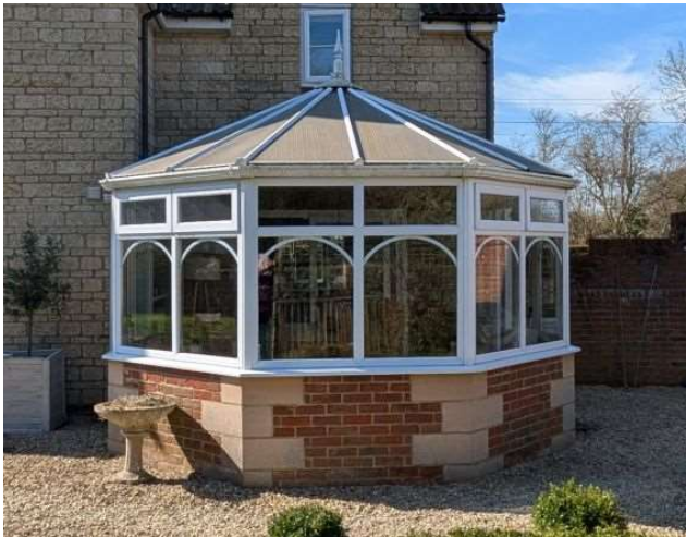
5 - Existing conservatory showing existing brick panels
