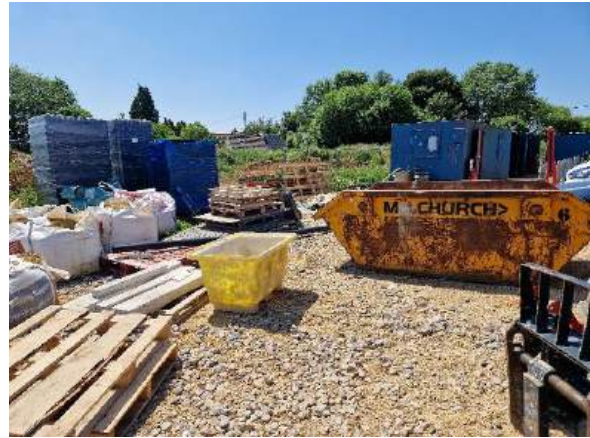
Photo 2. Parking and storage area in the north of the site (18 th June 2025).
