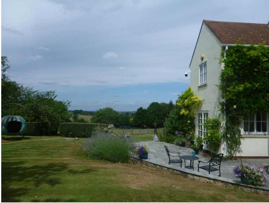
Fig 4: An area of patio to the west of the house will be affected by the extension.
