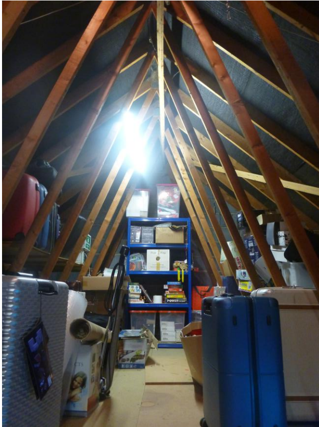
Fig 6: The loft space of Field House is boarded and used for storage. The roof is lined with bitumen roofing felt.
