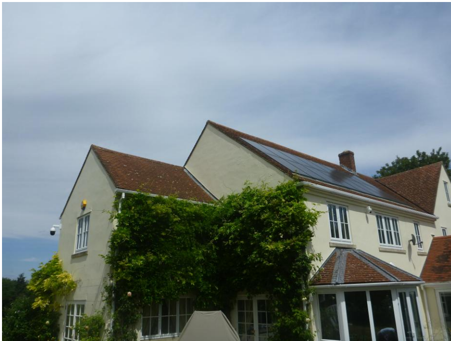
Fig 5: The roof and walls of Field House support no gaps or crevices.
