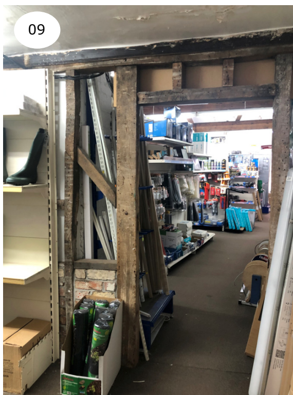
Partition on First Floor revealing Timber Frame Construction
