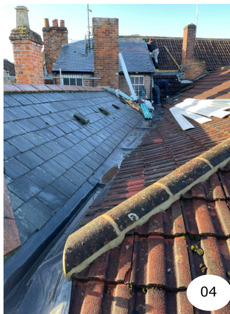
Maintenance work to roofs shared by 12 & 13 Maryport Street
