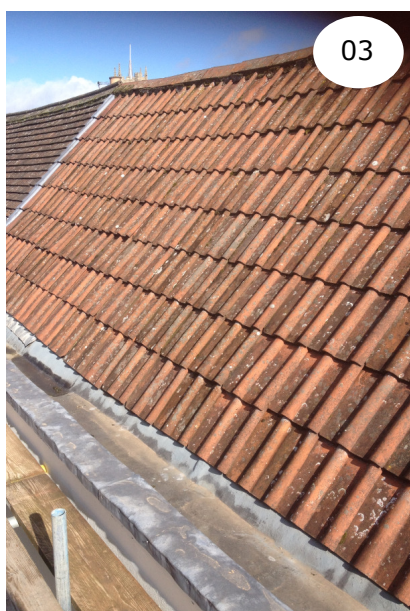
Recently repaired roof facing Maryport Street
