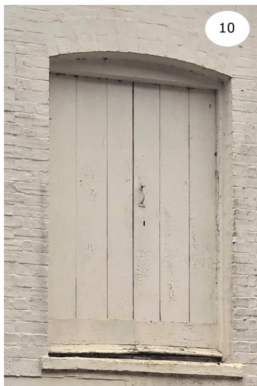
Existing Sack Doors facing Monday Market Street
