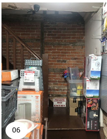
Existing Staircase First – Second Floor
