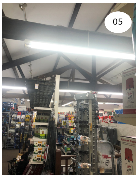
Roof Trusses visible at rear of First Floor
