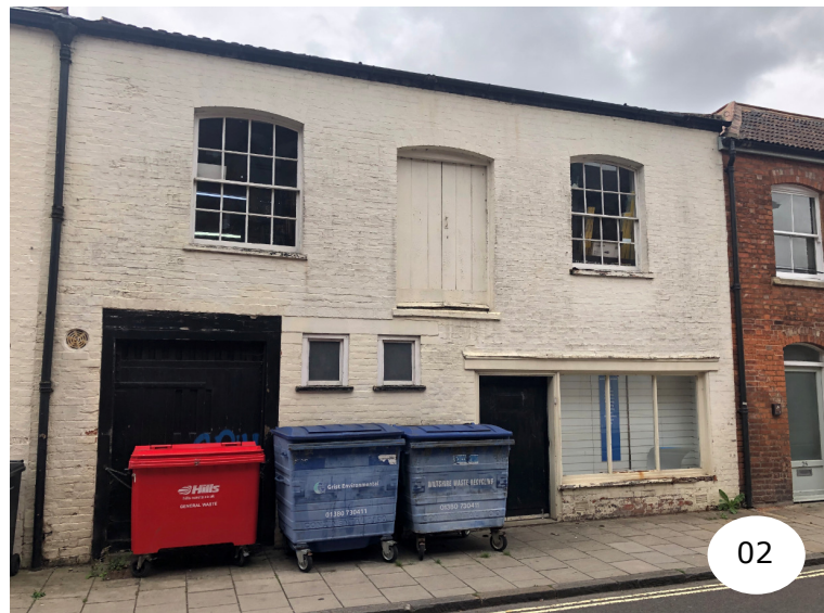
Rear Elevation facing Monday Market Street
