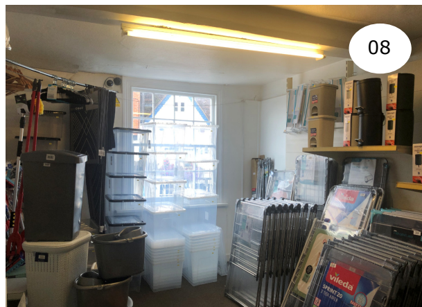
Partition between First Floor Rooms facing Maryport Street
