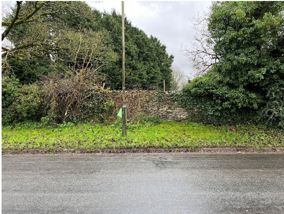
Plate 1: Potential curtilage-Listed dry-stone wall along the Easton Town boundary of the application site.
