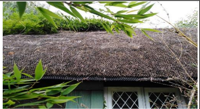
Photograph 2. View of thatched roof completely covered in chicken wire.
