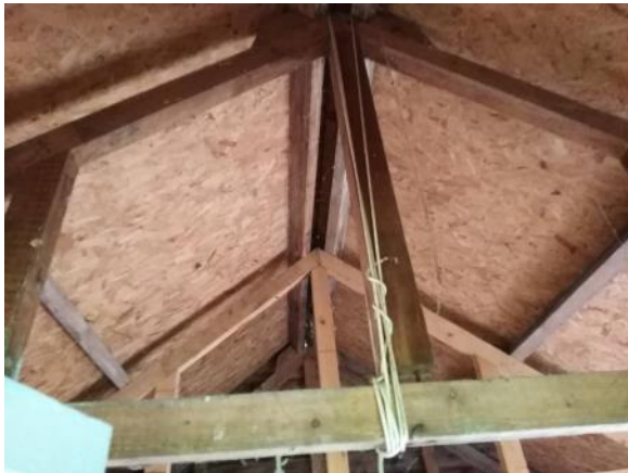
Photograph 7. View of the well-sealed internal building.
