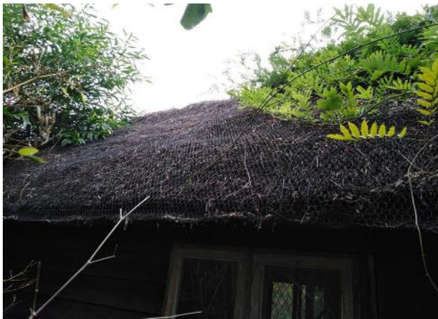
Photograph 3. View of thatched roof completely covered in chicken wire.
