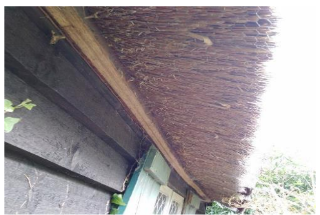
Photograph 6. Further views of the underside of the eaves and thatched roof.
