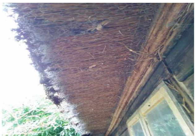
Photograph 5. Another view of the underside of the eaves and thatched roof.
