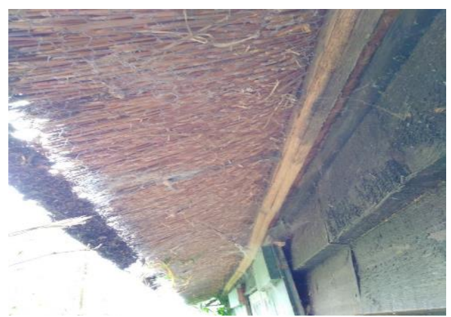
Photograph 4. View of underside of eaves and thatched roof.
