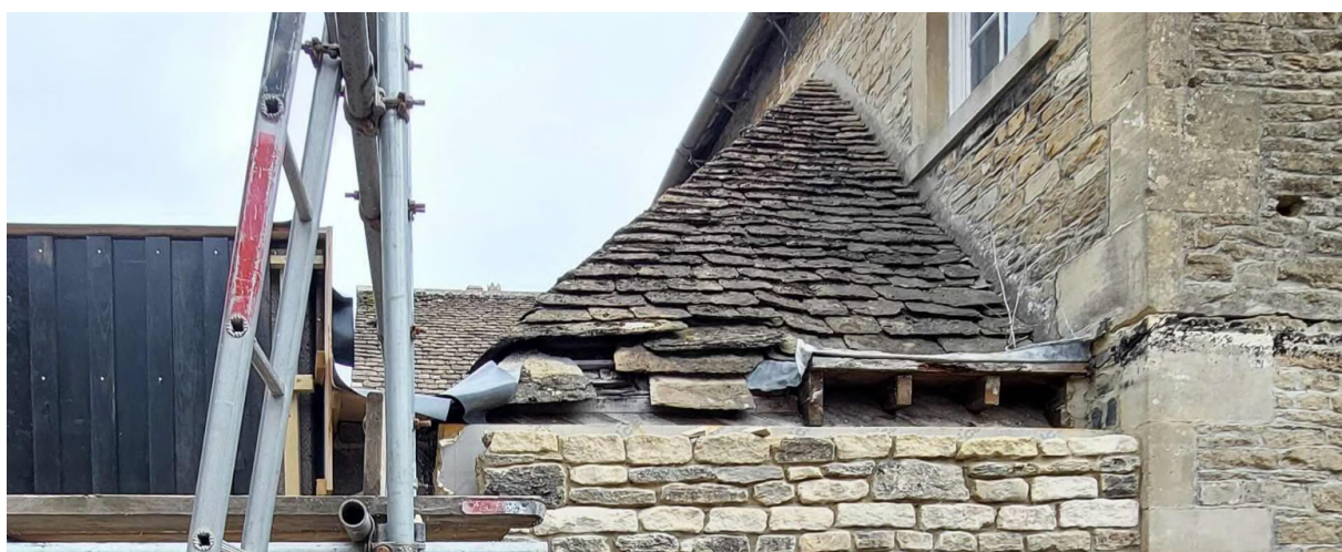
Remains of ATM extension flat roof structure still to be removed at right, with area of missing stone roof tiles at centre where part has been removed, above re-instated stone wall below. Approved vertical timber cladding of new kitchen extension at left rising to hide roof level ductwork on flat roof behind.
