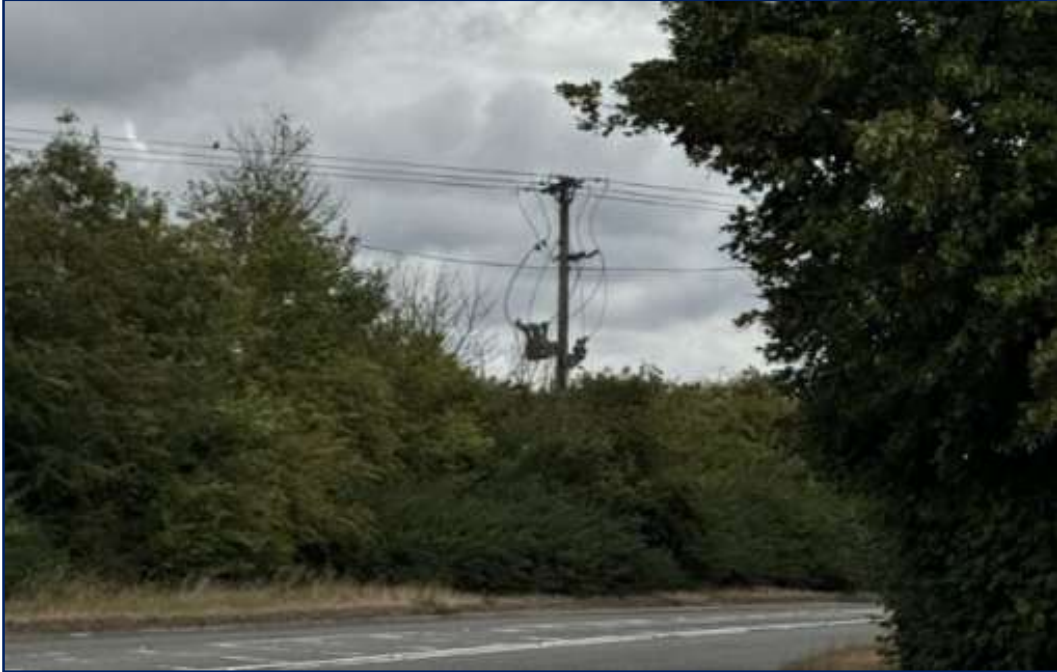
Figure 4: Image of existing PMCB
