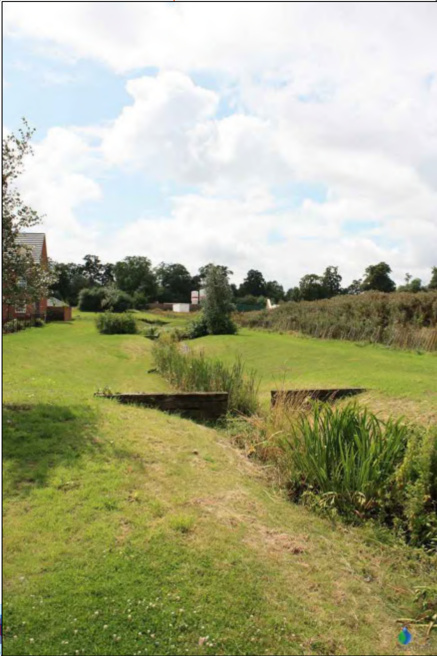
Figure 2: Example of a swale (Susdrain, July 2012).
