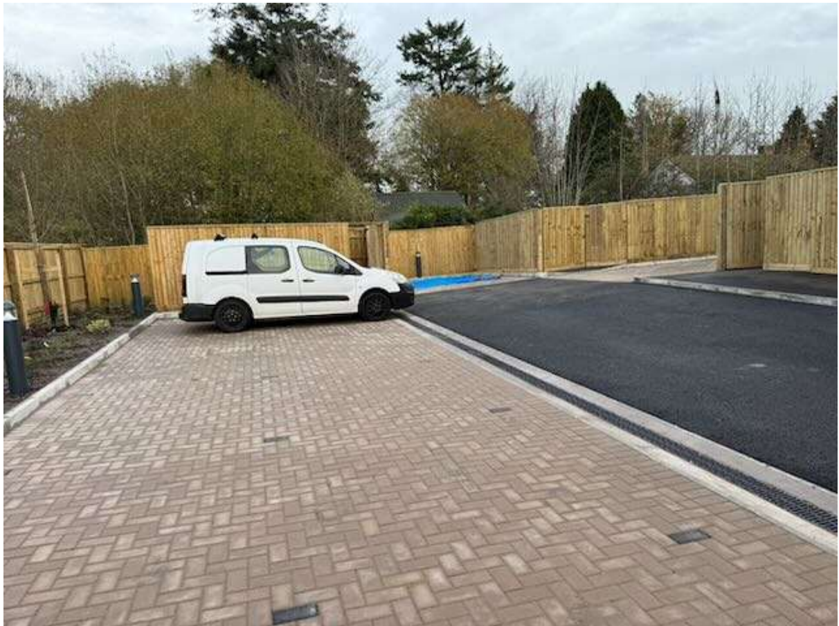
The parking spaces at the eastern end of the site.
