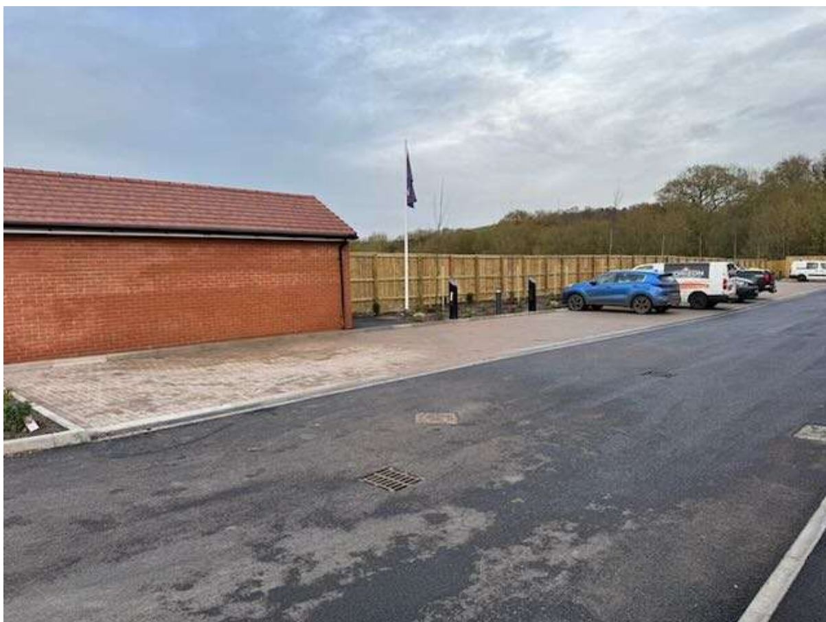
The main row of parking spaces along the northern boundary of the site.
