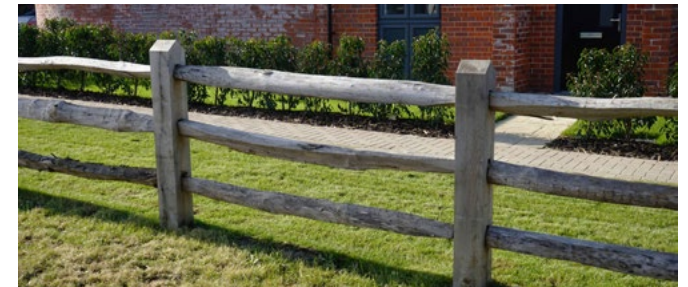
Cleft post and rail fencing precedent
