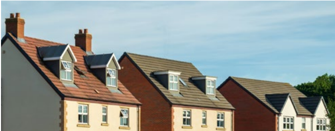
Visual interest in the roofscape created by chimneys, dormers with differing roof pitches and gable fronts
