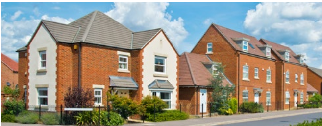
Corner turner with accent material and brick quoins on gable fronts
