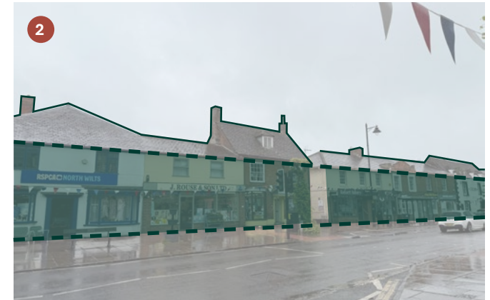
Variation in roof pitch, form and detail combined with a consistent two-storey frontage
