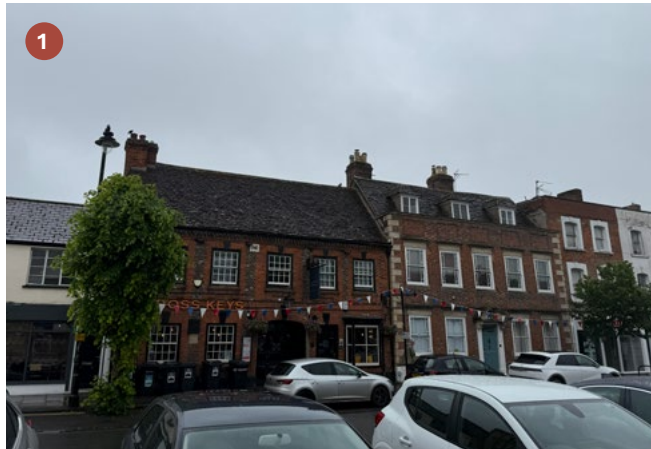
Regular window placement across building façades
