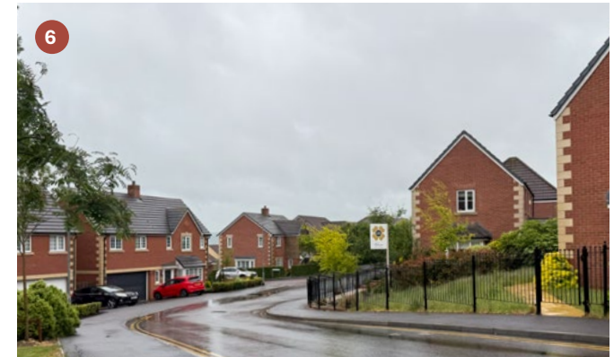
Chimneys and front gables create variety within the roofscape. Stone quoins and window dressings add visual interest to the streetscape
