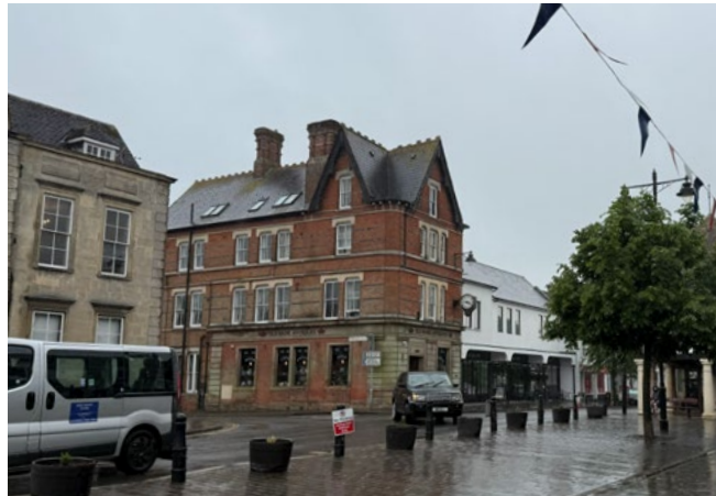
Remaining landmark building from The Royal Oak Hotel
