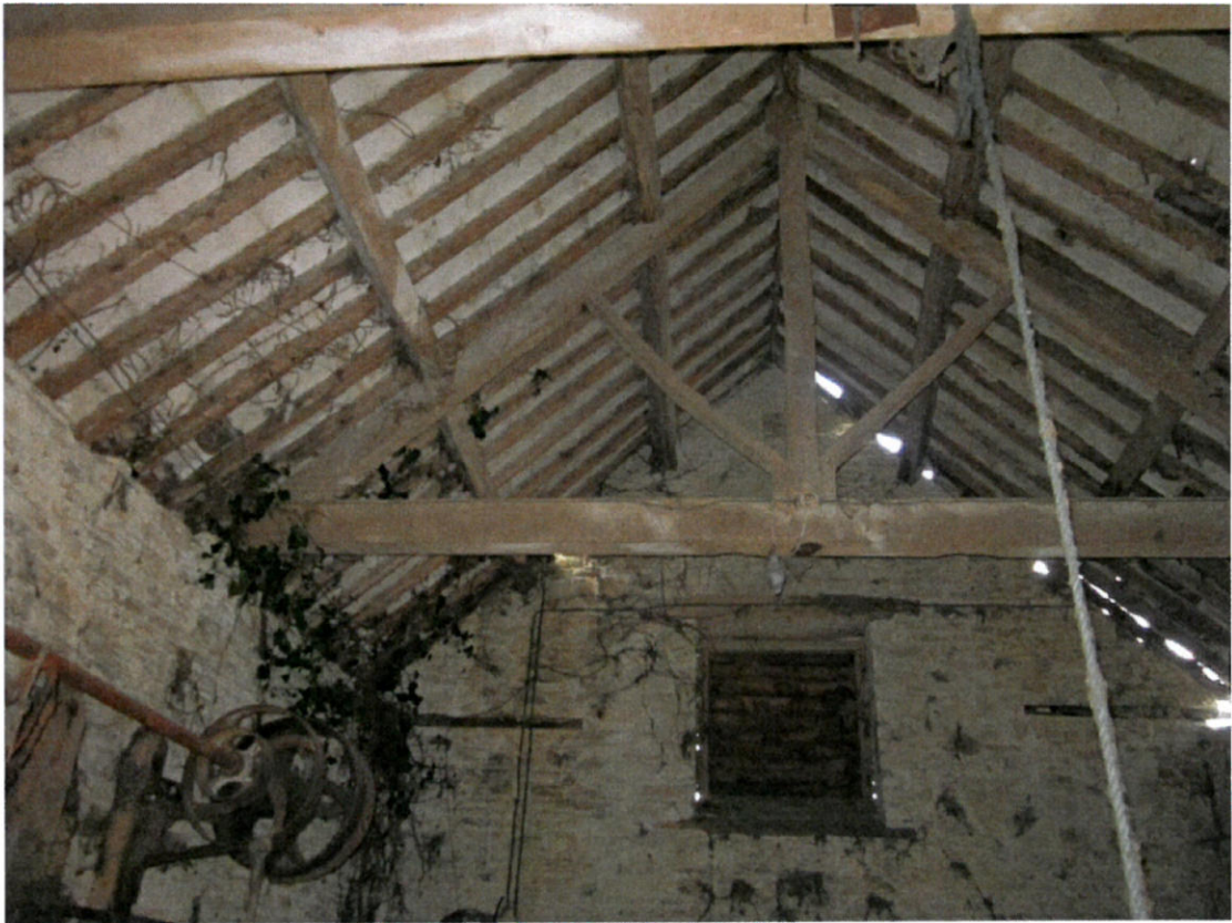
No: 5 Barn 4 - Roof Structure
