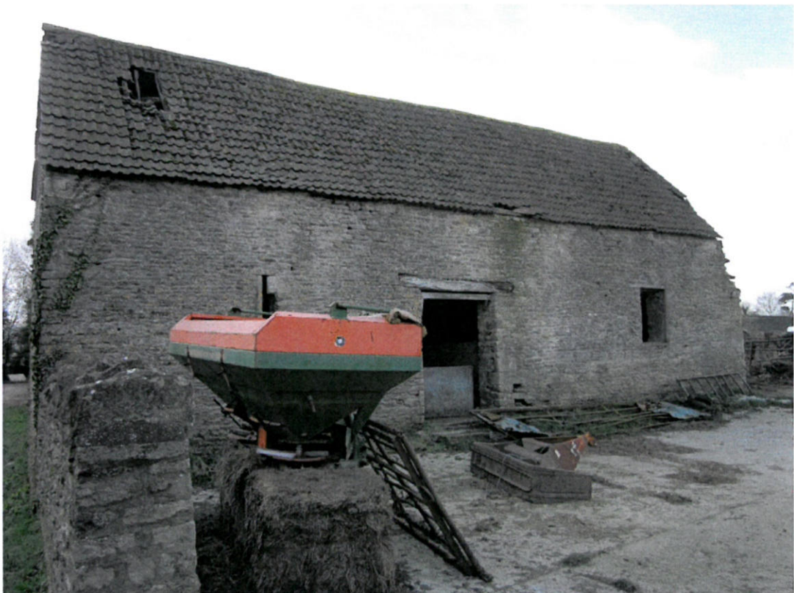
No: 2 Barn 4 - Rear Elevation
