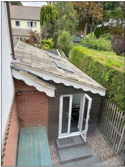
04 -As built aerial of extension, roof and rooflights
