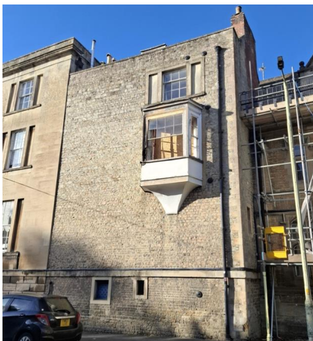
Photo (i) – elevation with oriel window
