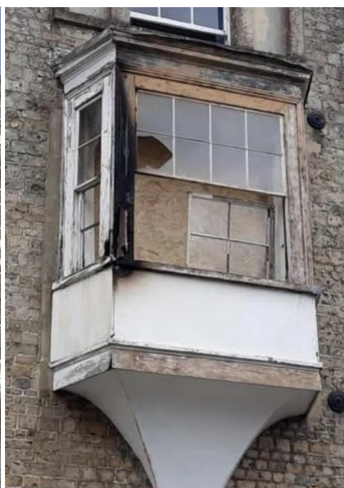
Photo (ii) – close up of oriel window
