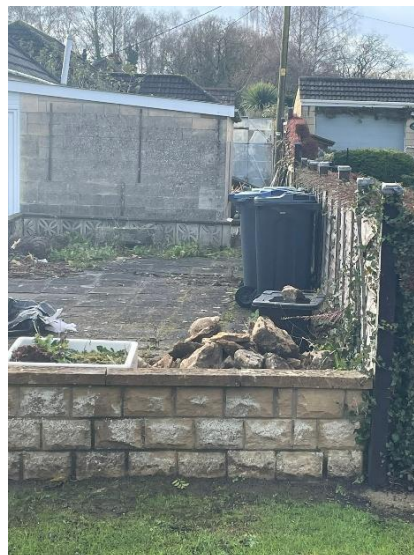
Elevation looking west boundary No.16
