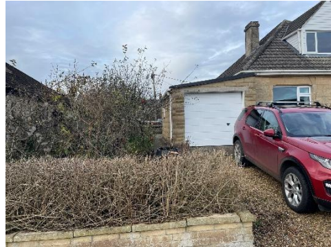
Boundary wall south elevation
