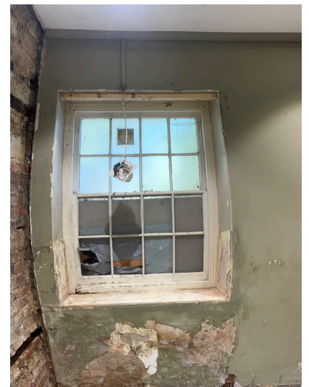
The condition of north elevation window.
