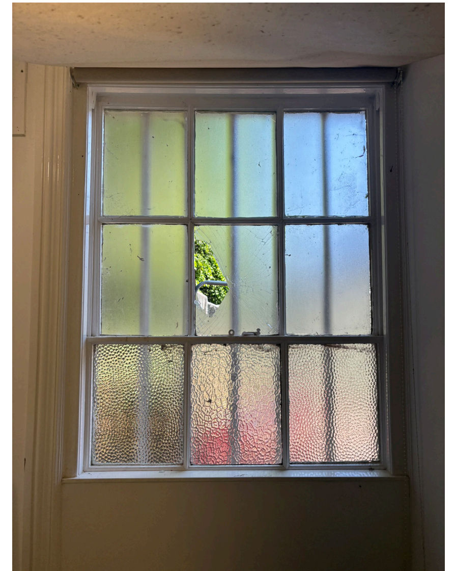
Existing window within north elevation of the WC
