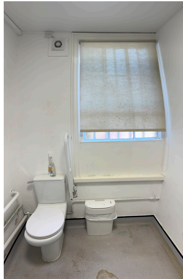
Existing north elevation of the WC
