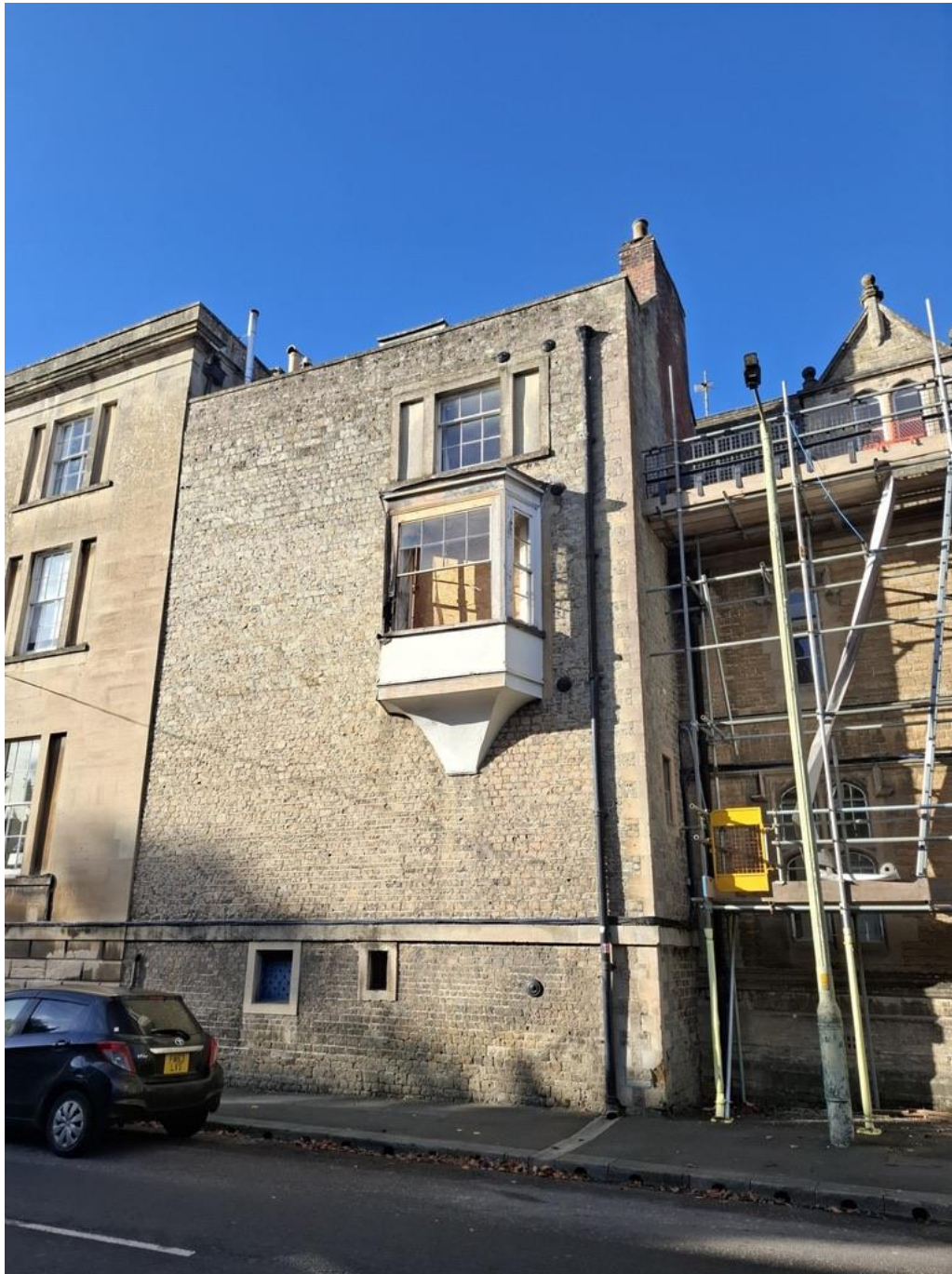
Photo (i) – elevation with oriel window
