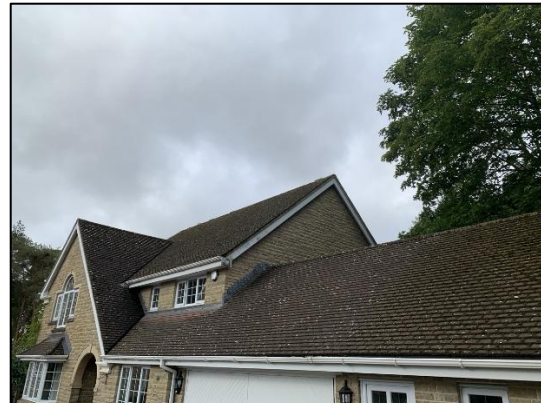
Photo 4 Side North elevation
