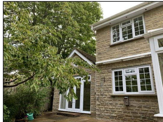
Photo 6 North West rear end of building
