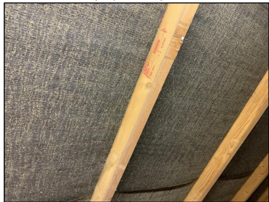
Photo 12 Internal roof of garage
