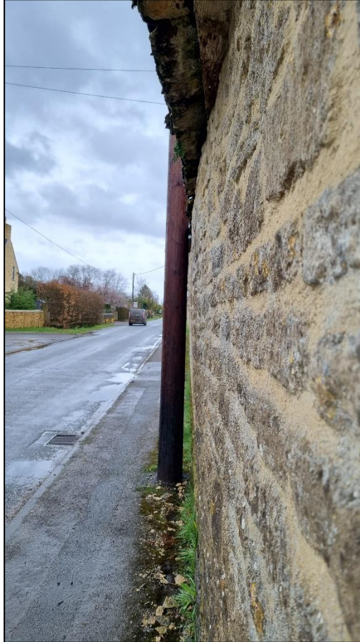
Photograph 10: Lean to rear wall
