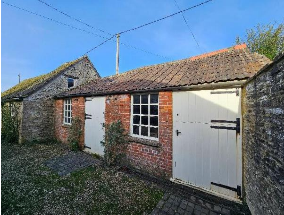
Fig.4 Smaller range – brick walling and triple Roman clay tiled roof
