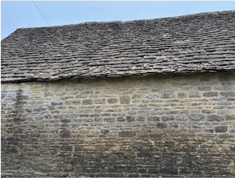
Fig.8 Natural stone tiles on the northern roof slope of the larger range
