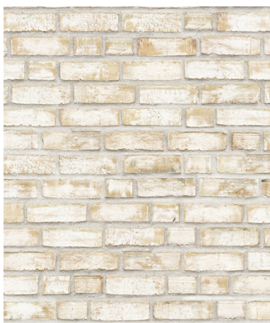
Buff Brick with Lime Mortar
