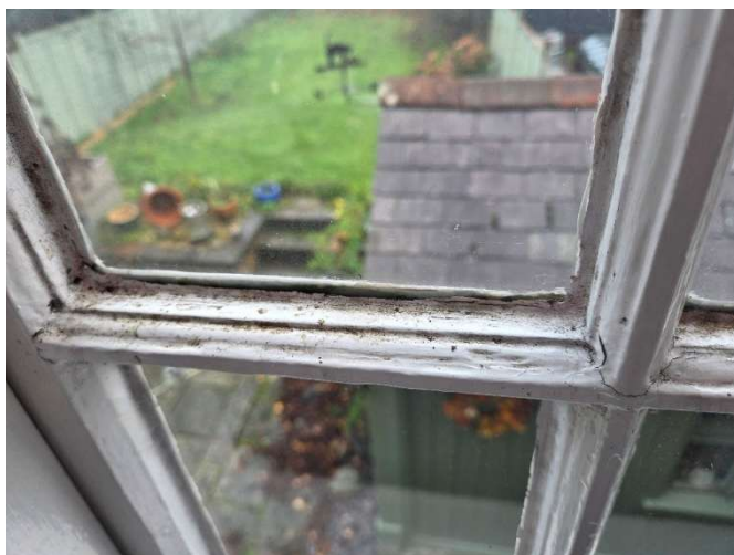
Photo to the right (W1) interior damage caused by condensation.
