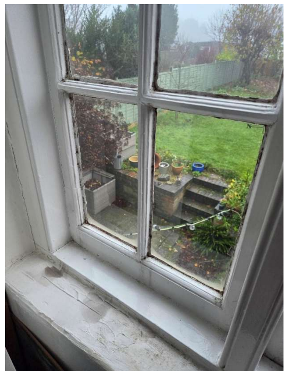
Photo to the right (W1) interior damage caused by condensation.
