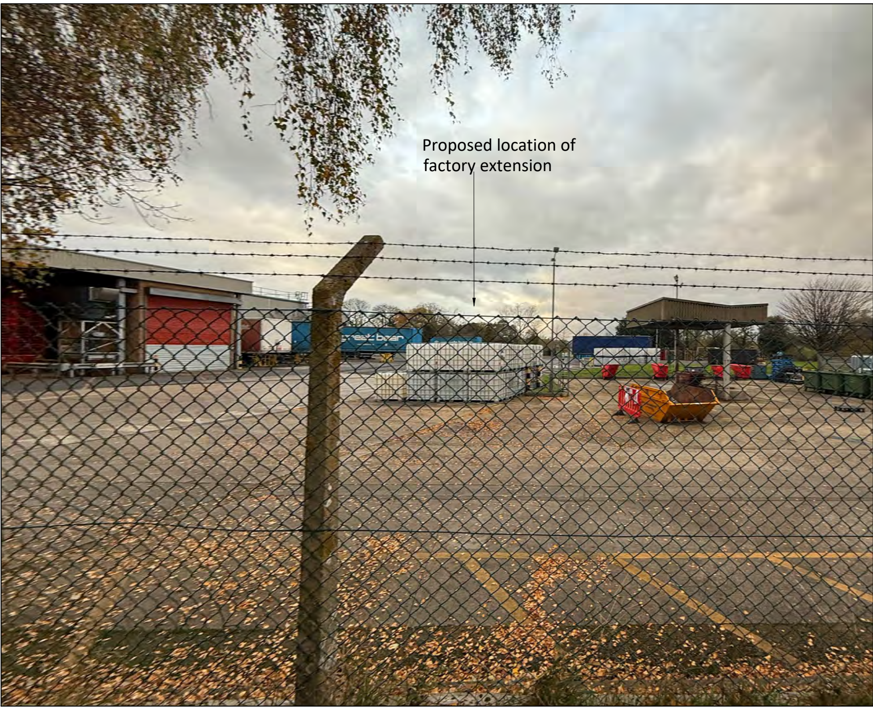
Viewpoint 6 from Stav1 right of way looking into factory extension site
