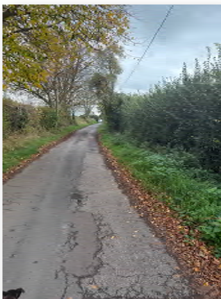
Image 1: Looking east along The Star Lane with sunken road and high hedgerows.
