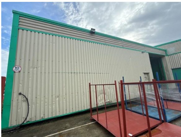
Photo 1 Southeastern storage facility (front)
