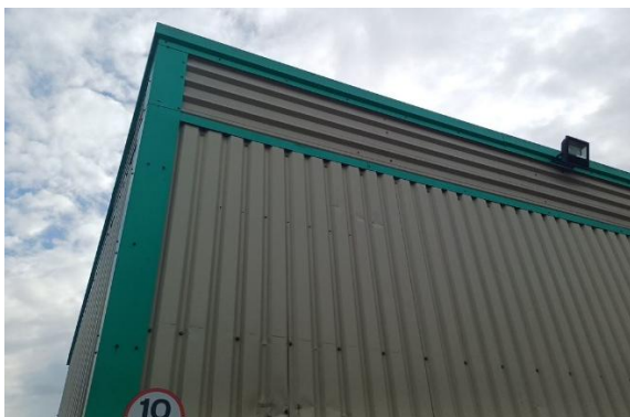
Photo 5 Exterior onsite storage shed (B1)
