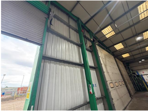
Photo 7 Interior wall offsite factory (B2)
