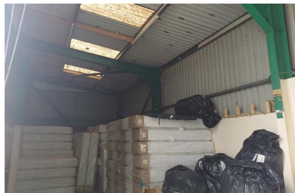
Photo 6 Interior onsite storage shed (B1)
