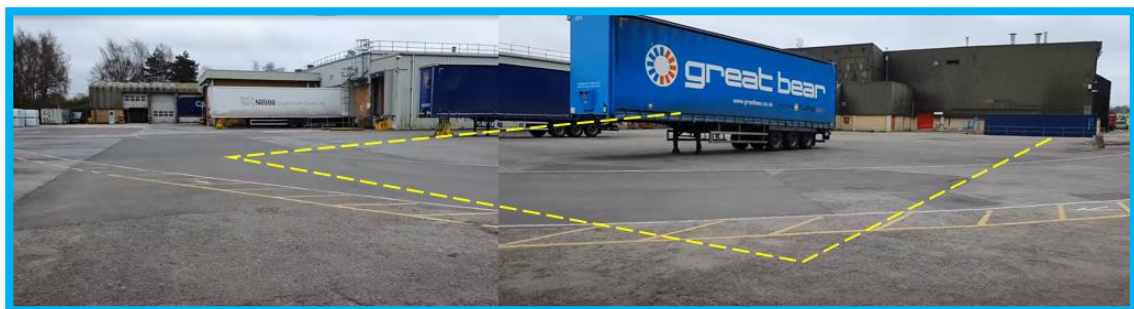
Figure 5 Panoramic image of existing site, with approximate outline of proposed factory in yellow broken line.
