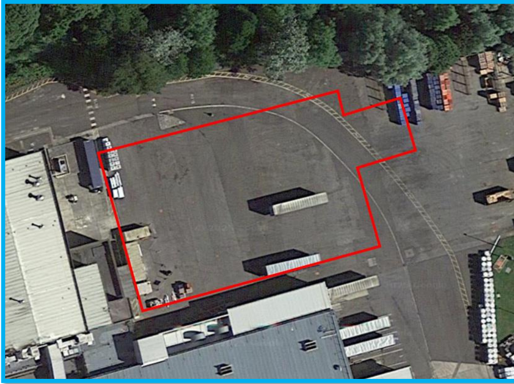
Figure 3 Location of Site on existing macadam and concrete service yard. (Google Earth).
