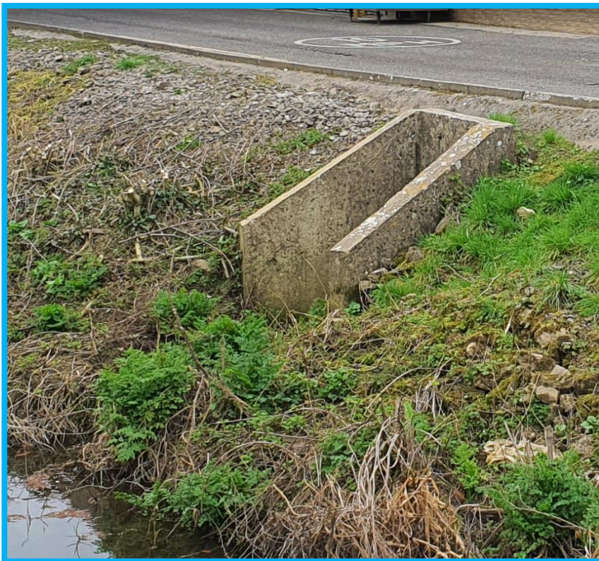
Figure 21 Existing headwall, typical of headwall at discharge point
