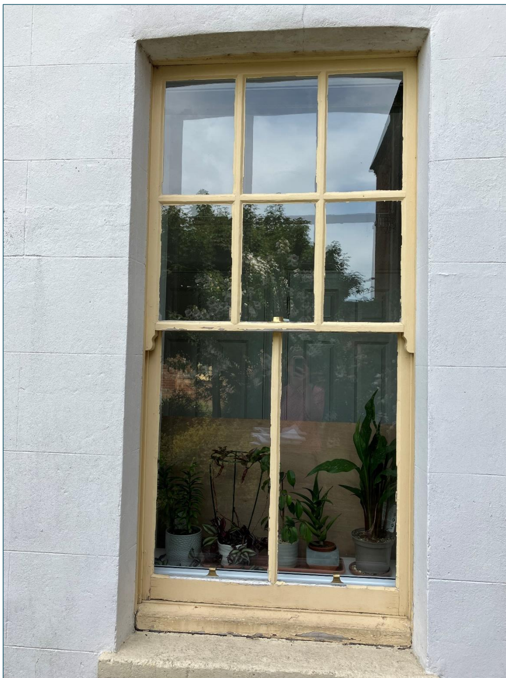
Figure 8 – Single glazed timber double hung sliding sash windows – six over two configurations with secondary glazed unit fitted to internal reveal.
