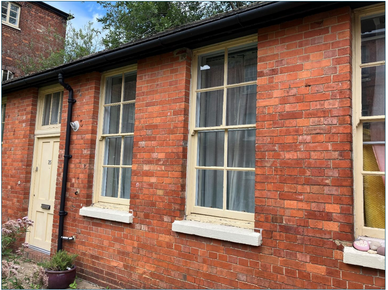
Figure 14 – Historic single glazed timber top hung sliding sash windows.
