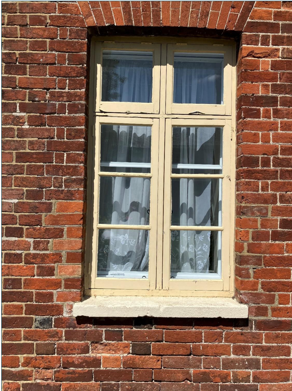
Figure 11 – Non-original single glazed top and side hung timber casement window with secondary glazed unit fitted to internal reveal.
