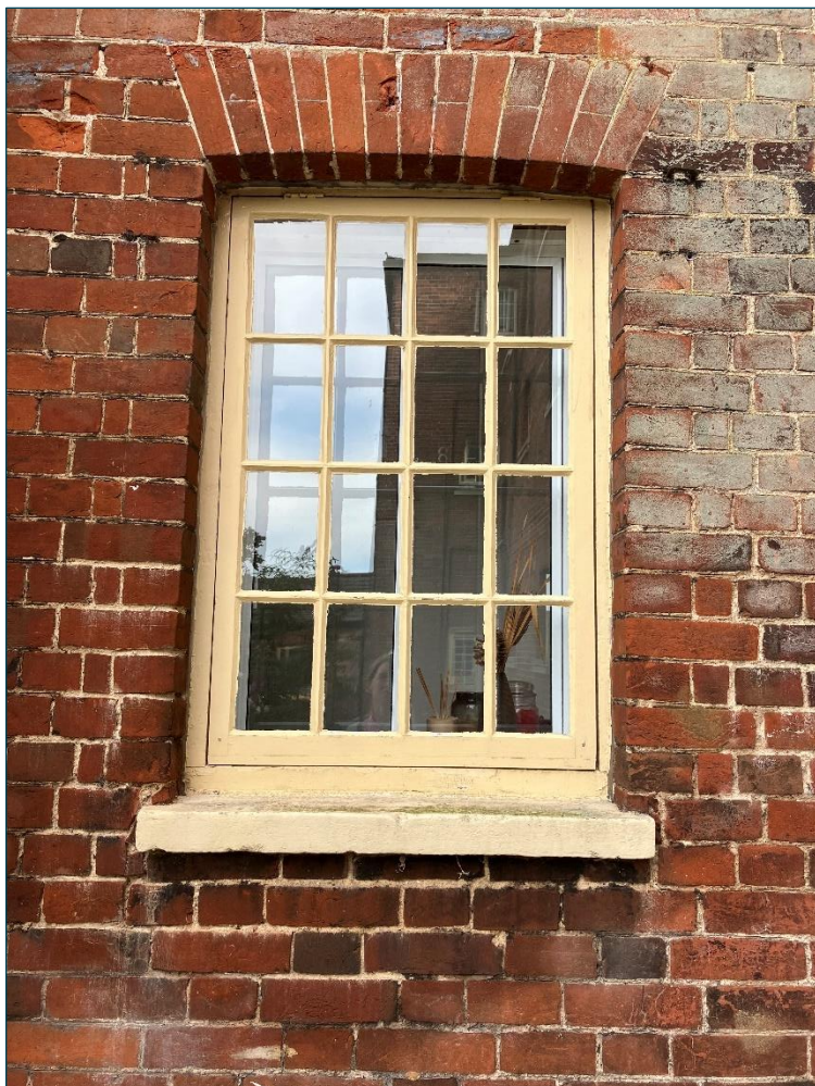
Figure 7 – non-original single glazed top hung timber casement window with secondary glazed unit fitted to internal reveal.
