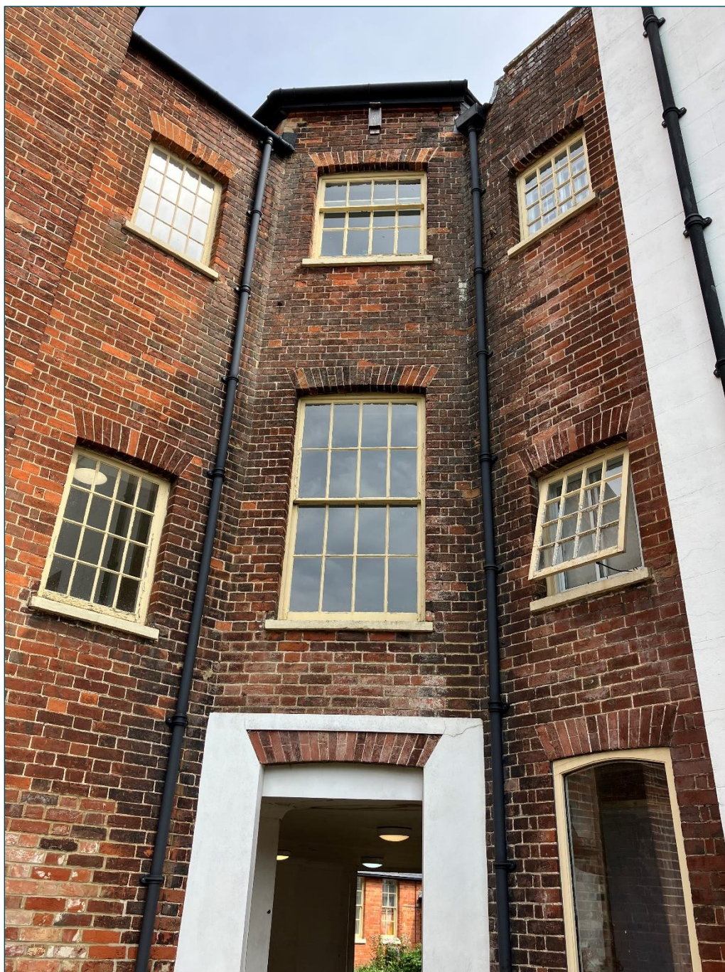
Figure 13 – Historic single glazed timber top hung sliding sash windows to octagonal cross point of wings.
