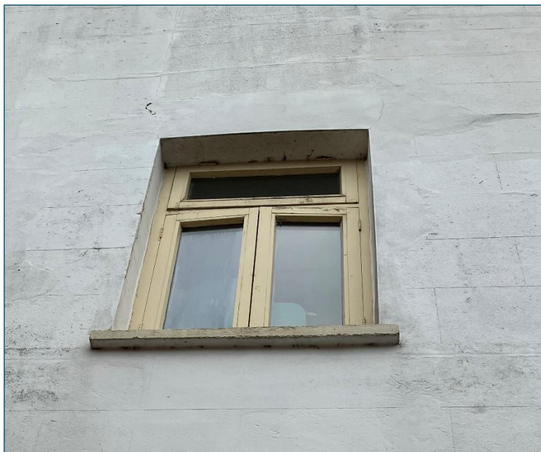
Figure 17 – Non-original timber single glazed casement window installed on main block, to be replaced with timber double glazed casement window in a style to match the wider scheme, incorporating glazing bars.
