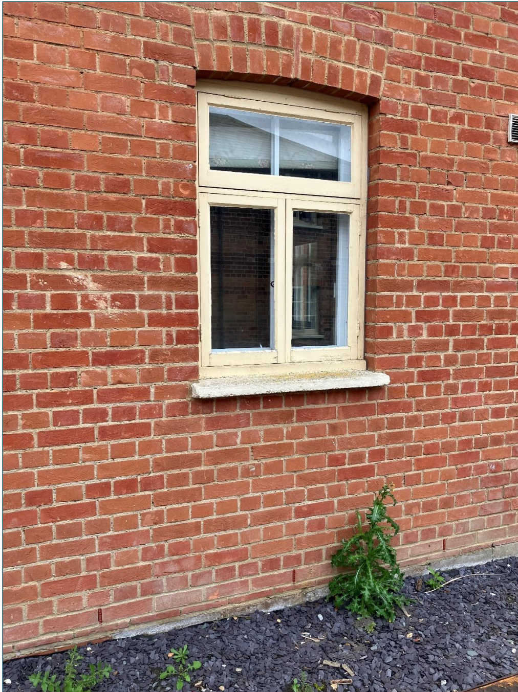
Figure 10 – Non-original single glazed top and side hung timber casement window with secondary glazed unit fitted to internal reveal.
