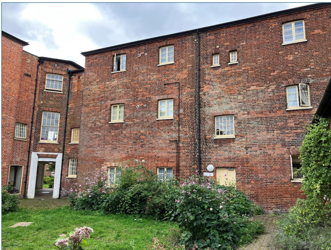
Figure 3 – Kingsway House (East Facing Elevation 2)
