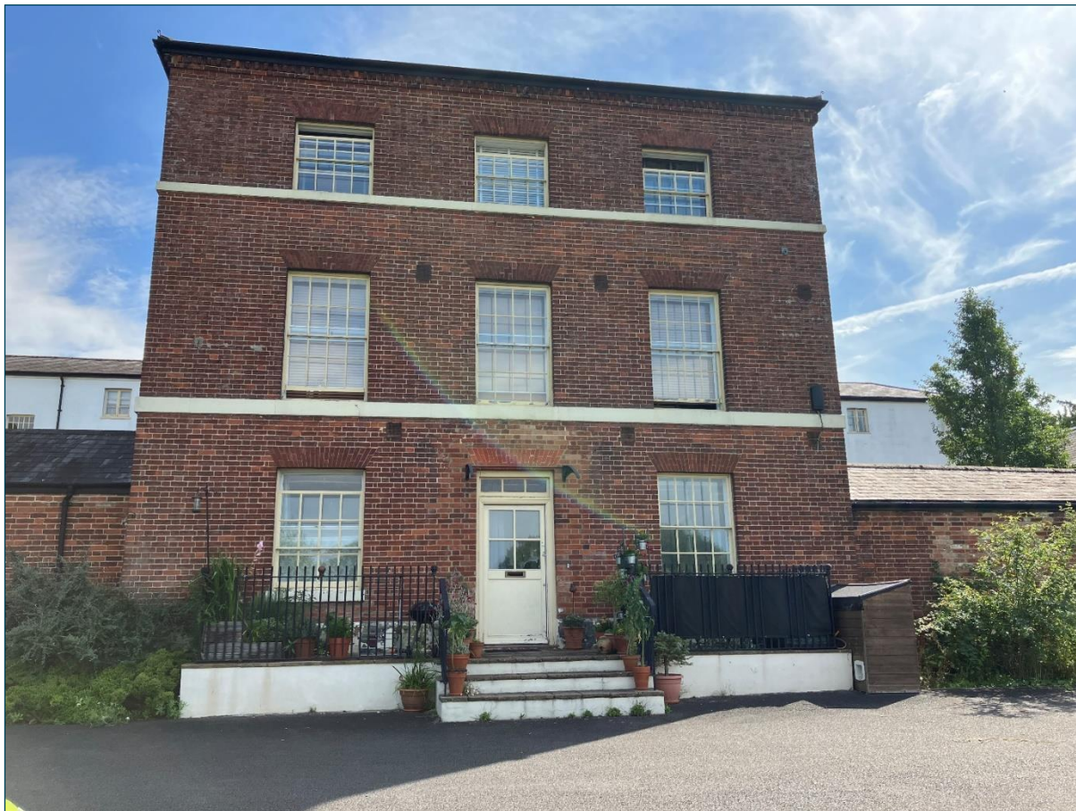
Figure 6 – Kingsway House (West Facing Elevation 1).
