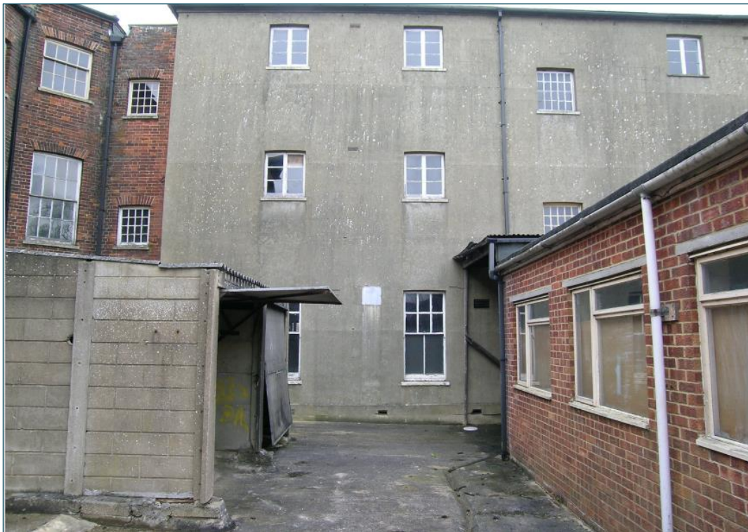
Figure 19 – West elevation prior to conversion to residential accommodation in 2007. Note style and arrangement of existing windows.
