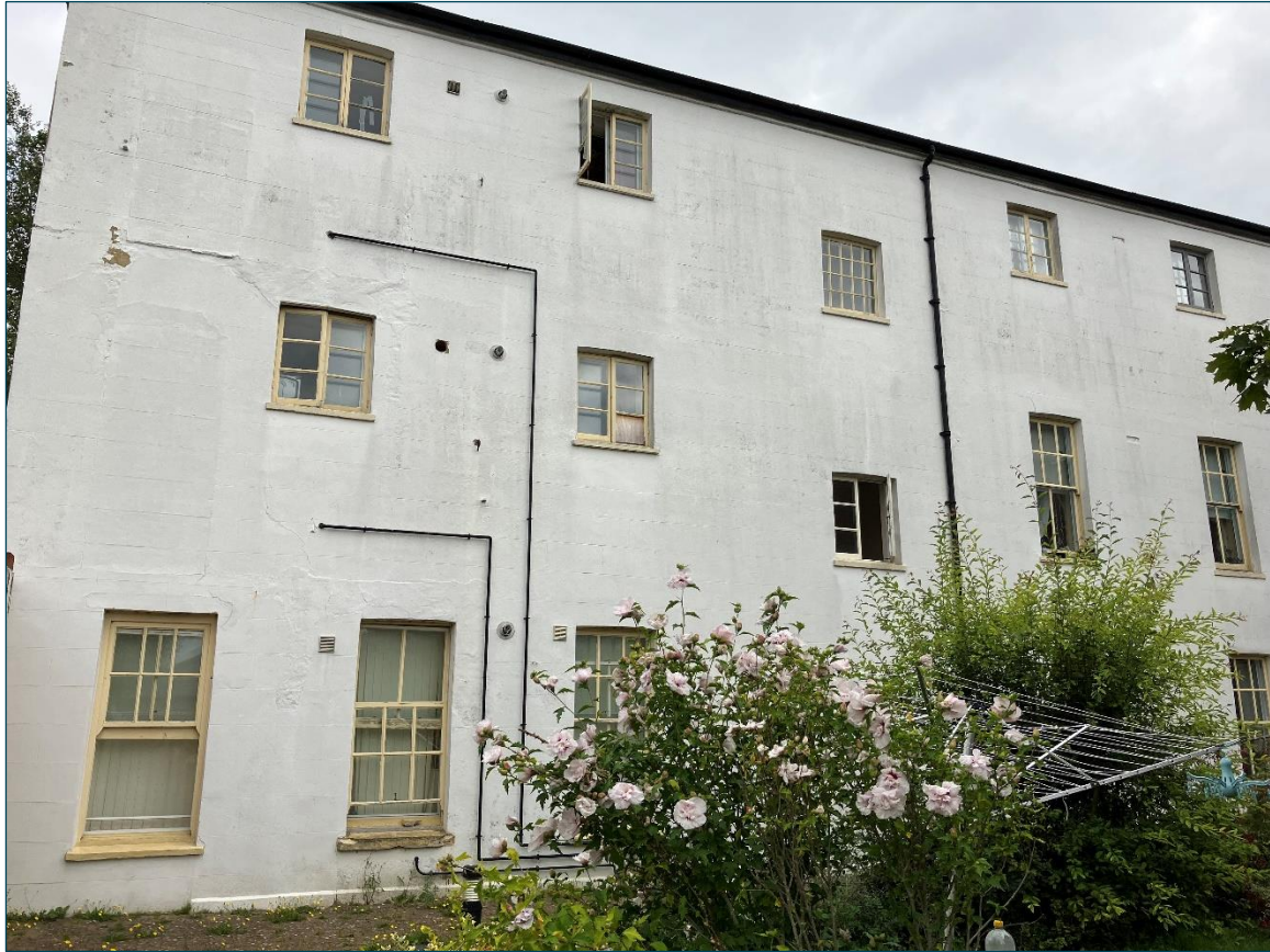
Figure 5 – Kingsway House (West Facing Elevation 2).
