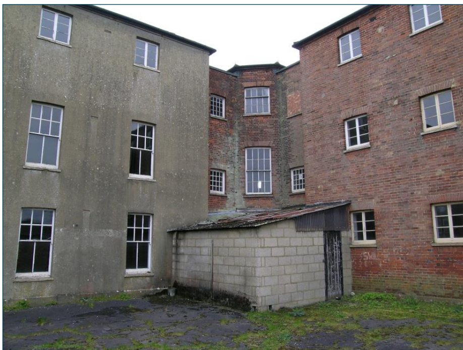
Figure 20 – West and North elevations prior to conversion to residential accommodation in 2007. Note style and arrangement of existing windows.
