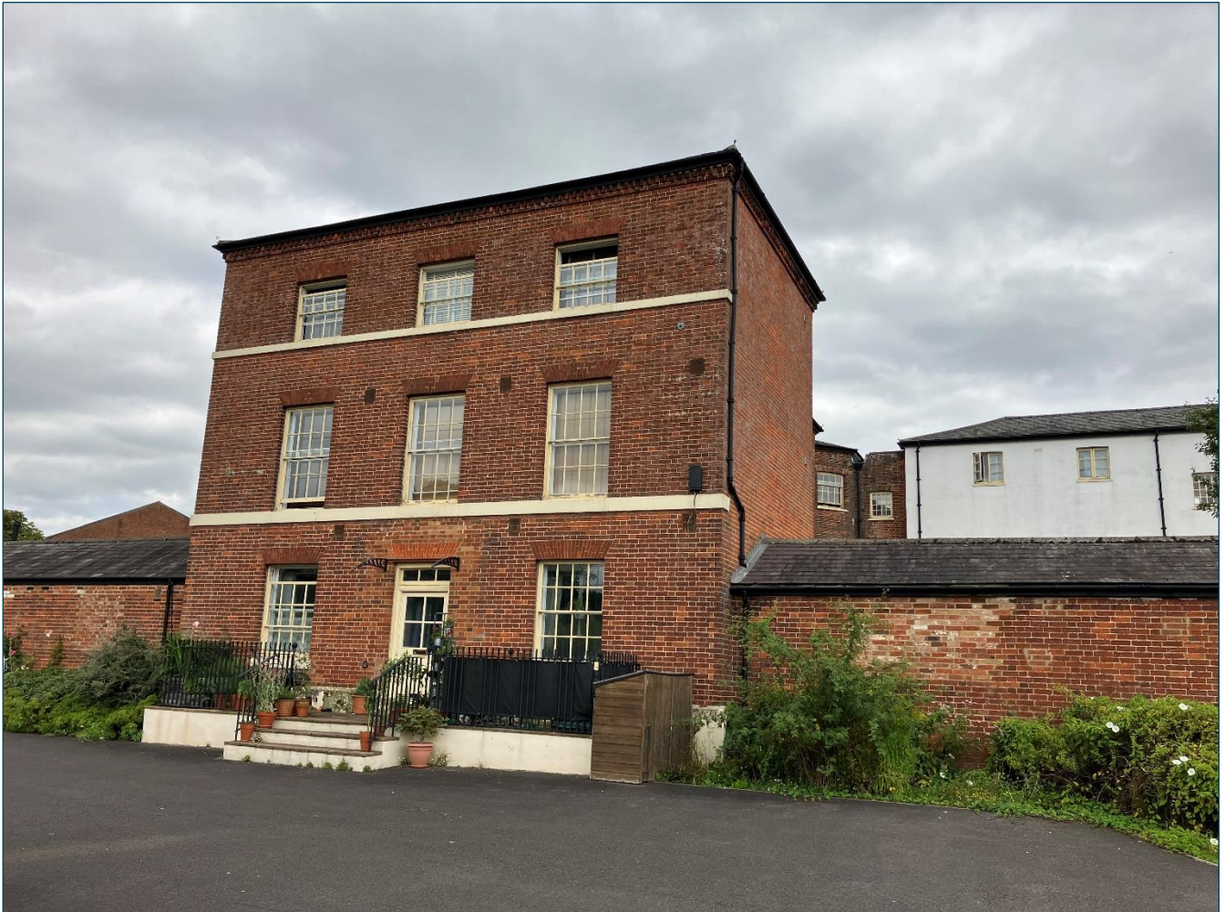
Kingsway House, Warminster Road, Wilton, Salisbury, Wiltshire, SP2 0FB – West Elevation
