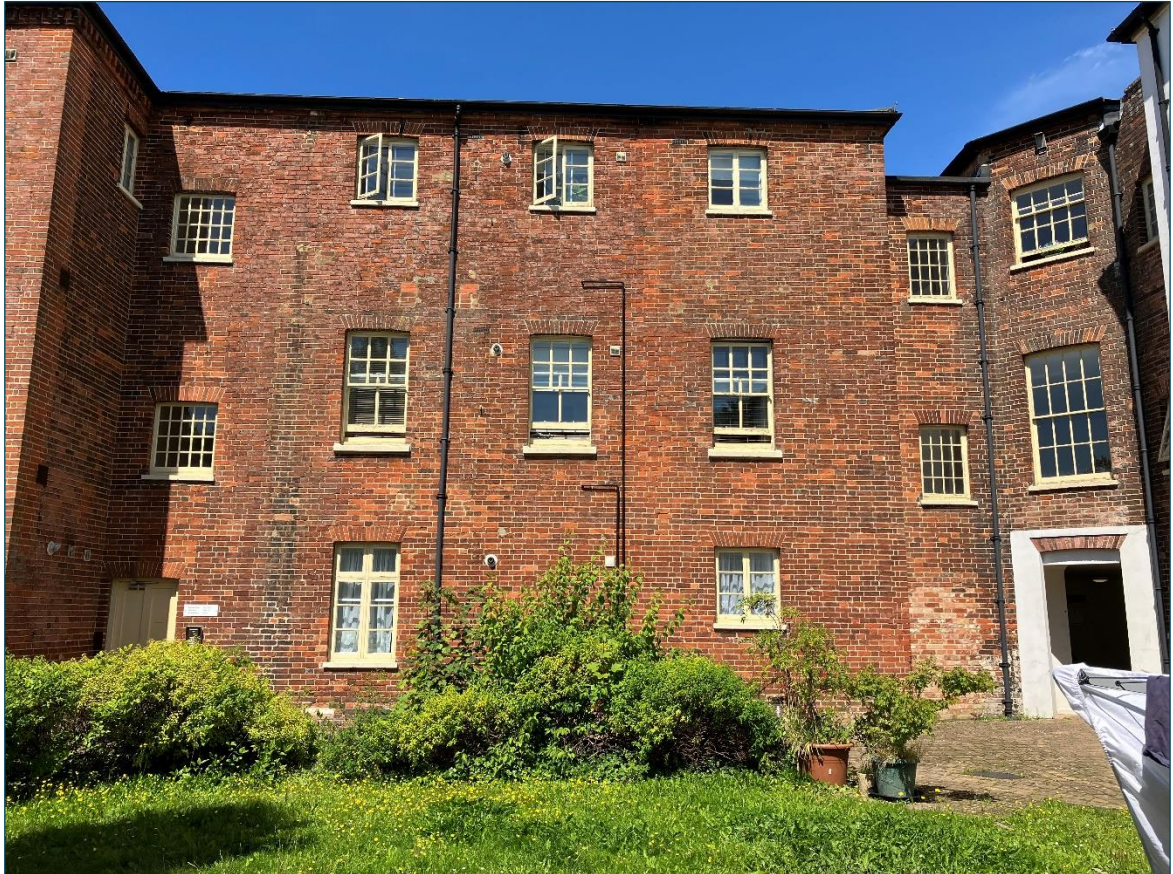
Figure 4 – Kingsway House (South Facing Elevation 2).
