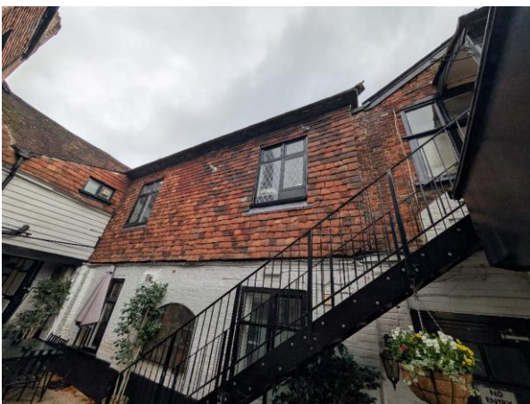
Photograph 5. Detail of hanging tiled section.
