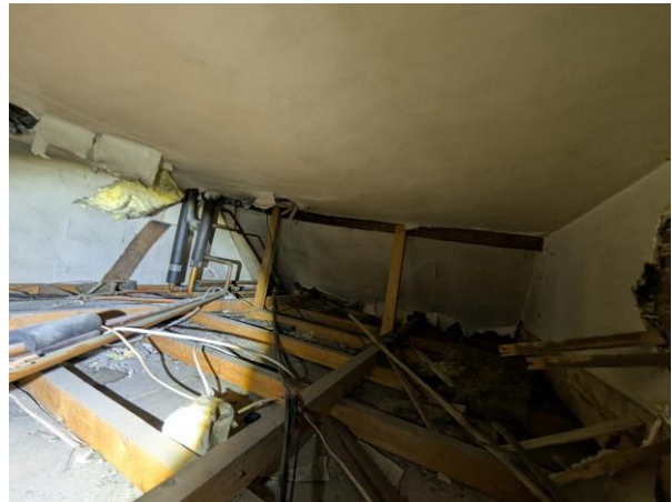
Photograph 10. Detail of loft space.
