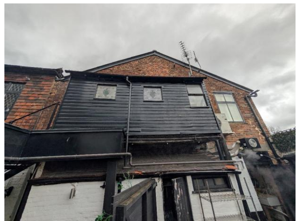
Photograph 6. Detail of wooden weatherboarded section.
