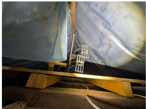
Photograph 12. Detail of loft space.
