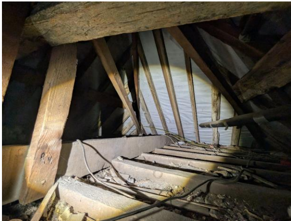
Photograph 9. Detail of loft space.
