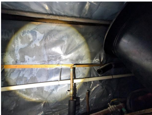
Photograph 11. Detail of loft space.
