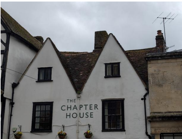
Photograph 3. Detail of the two gables to St John's Street.
