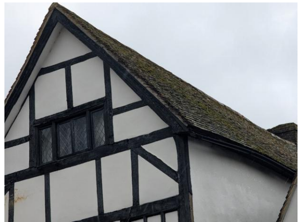
Photograph 4. Detail of the timber-framed gable to St John's Street.
