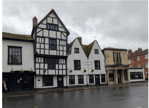
Photograph 2. General view of The Chapter House
