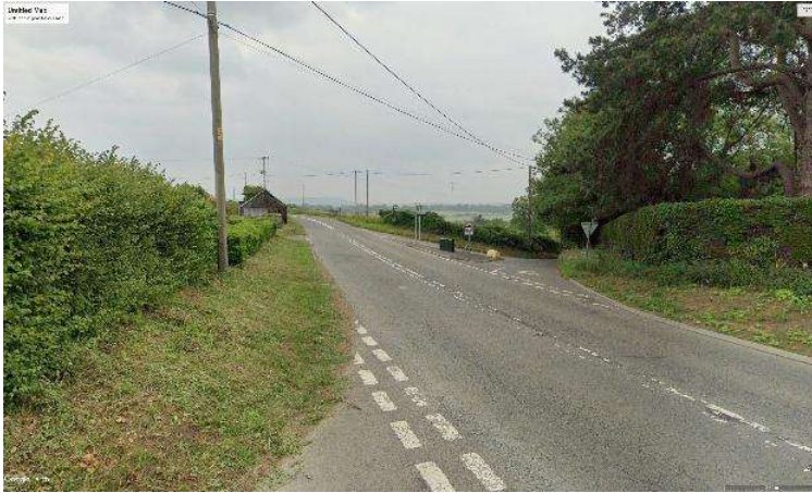
View, looking east along the A3102 at the junction with Sandridge Lane.
