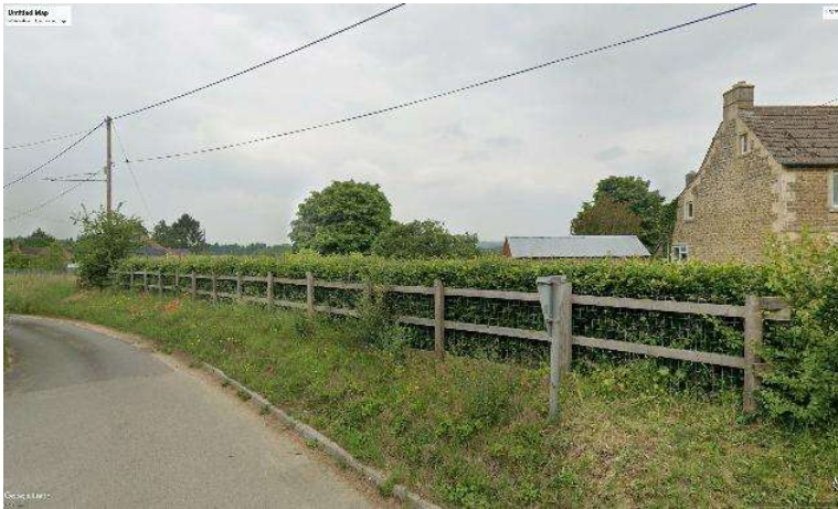
View, looking north along Sandridge Lane, showing the post & rail fence where the new access would be formed into the garden of Wilds Farm on the right.
