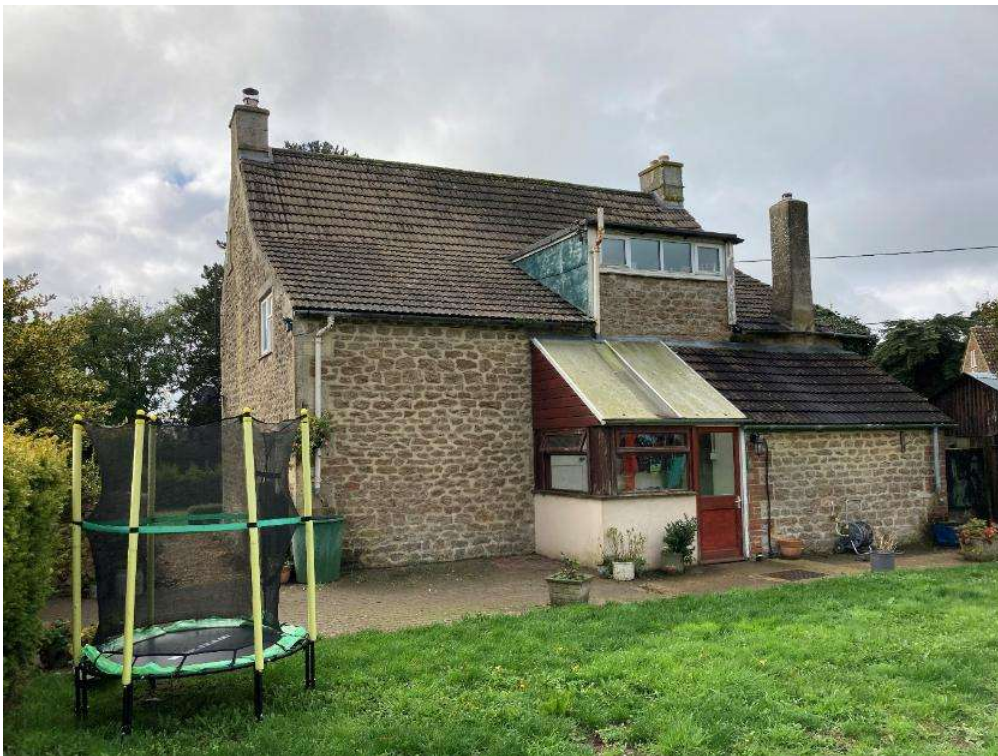
View of the rear, (north) elevation of Wilds Farm, from the north-east.
