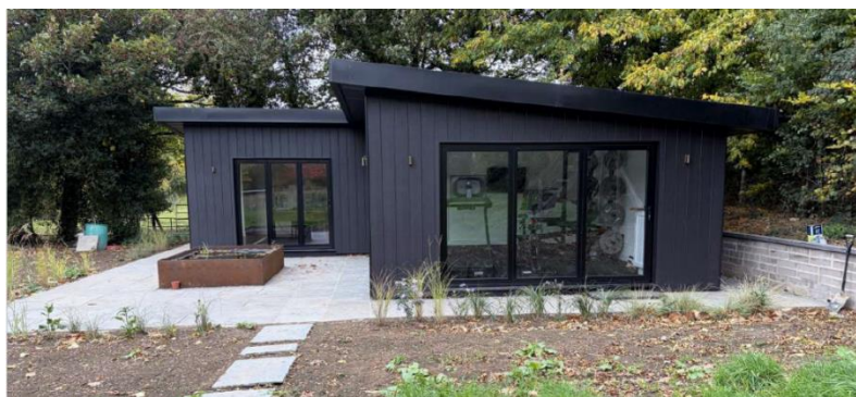
Photograph of Outbuilding
