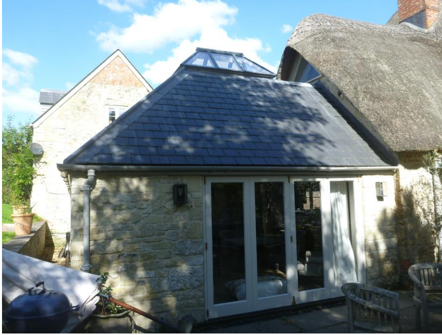
Fig 2: The more western extension to Stop Farm has a slate roof with a glazed portion at the ridge.
