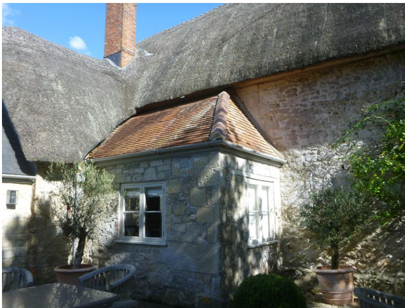
Fig 5: The other extension has a clay tile roof.
