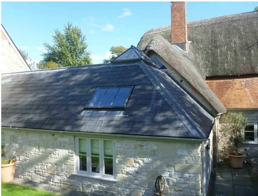
Fig 3: The slate roof of the western extension is tightly sealed.
