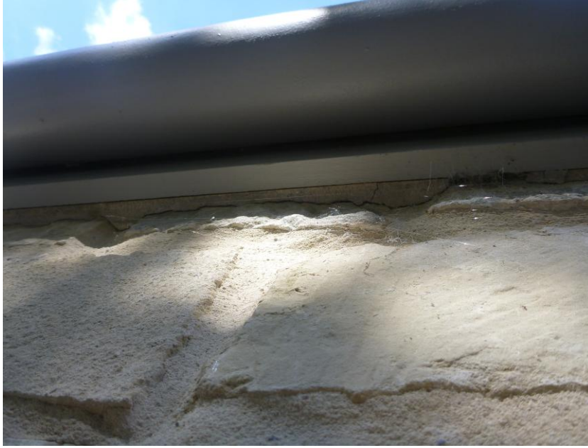
Fig 6: The eaves of the smaller extension are well sealed.
